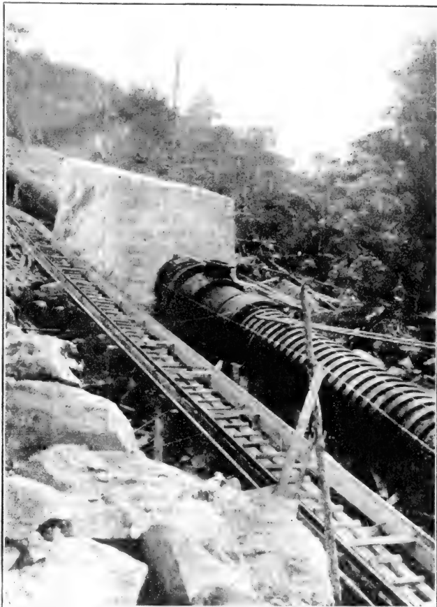
FIG. 1. - Large pipe welded by water-gas method. From Transactions of the Institution of Engineers and Shipbuilders in Scotland.
