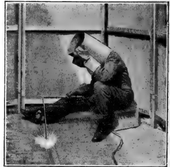
FIG. 2.—Repairing a tram-rail by arc welding, using an iron electrode.
