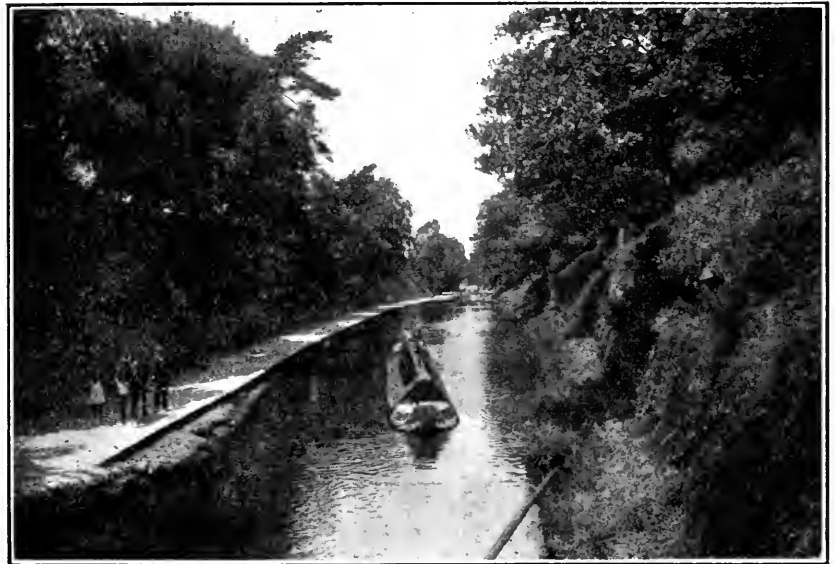
FIG. 2.—Canal in sandstone cutting. From "Practical River and Canal Engineering."
