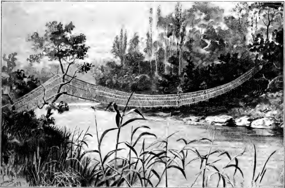
FIG. 1.—Native suspension bridge across the Vanapa river.
