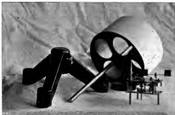
FIG. 1.—A Drum Recorder dismounted to show its parts.
