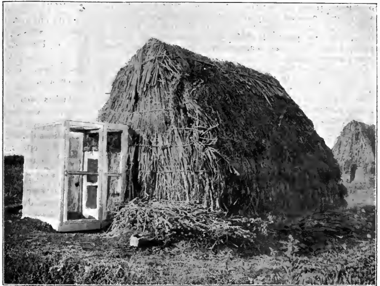
FIG. 2.—Hut with mosquito cage round door, which is itself mosquito proof (as suggested by Celli). Reproduced from a photograph lent by the Sanitary Institute.
