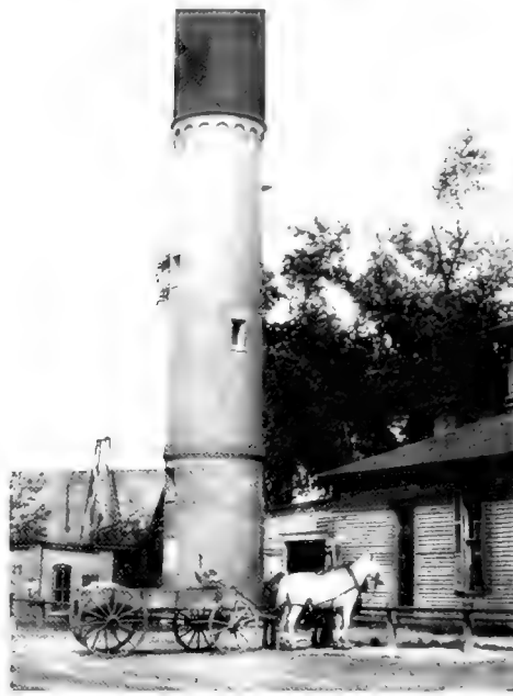
Water from wells was pumped into the concrete covered collecting reservoir and then filtered and treated at the Dwight Water Plant, c.1914. (Courtesy ISWS)
