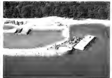
The City of Lake Forest is in the process of building an offshore breakwater to lessen the erosion along its shoreline. This is controversial since it may have adverse effects on property down the shore.
