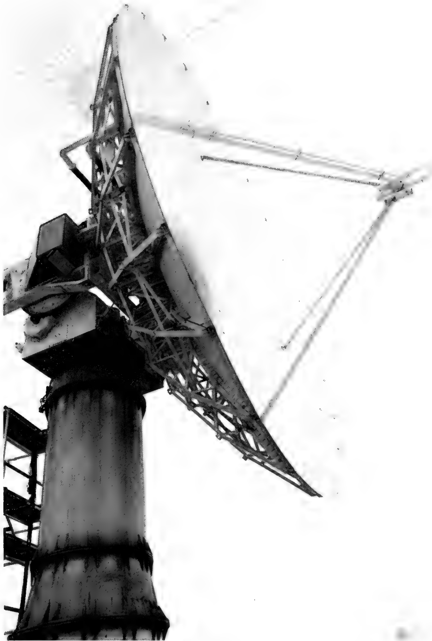
Antenna and pedestal of the CHILL radar system. The massive radar is 40 feet high and the antenna "dish" is 28 feet in diameter.
