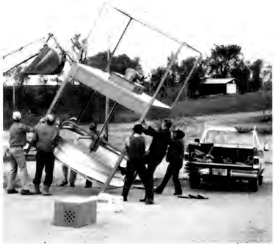
Lake Eureka destratifier prior to its installation.
