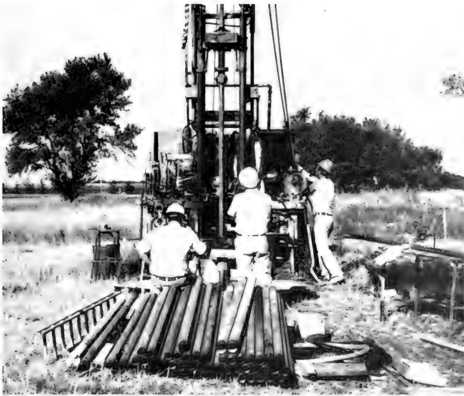
Geological Survey staff drill test holes for Illinois' proposed SSC site near Fermilab
