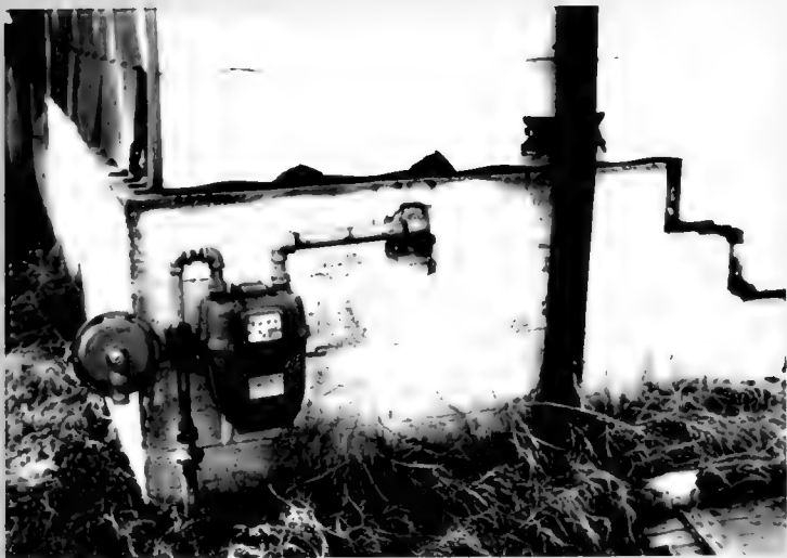
Mine subsidence damaged this home built over an old abandoned coal mine. Old room-and-pillar mines removed much more coal than today's regulated mine designs. (Courtesy: IGS)
