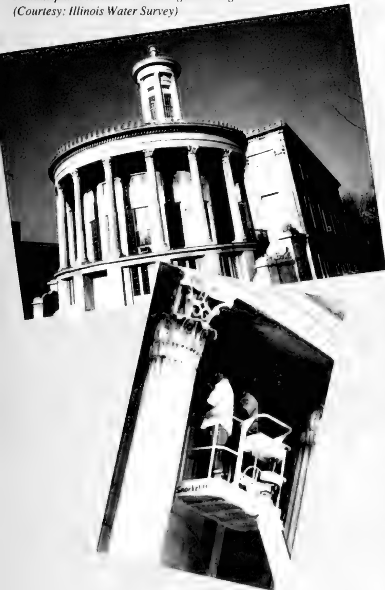
Saving a landmark (Courtesy: Illinois Water Survey)
