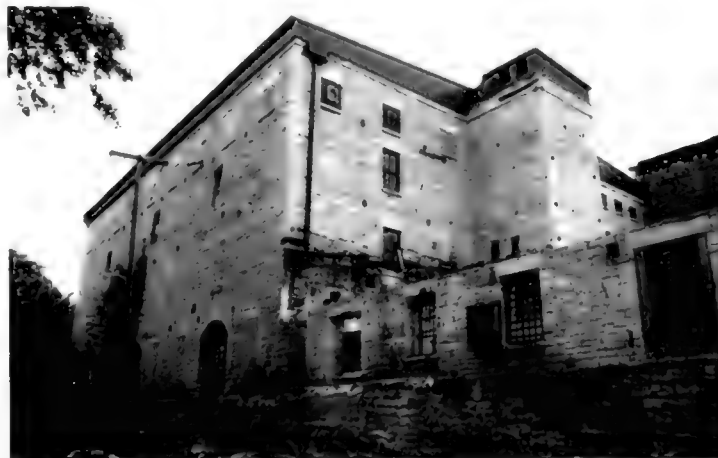
Norton Warehouse, Lockport
