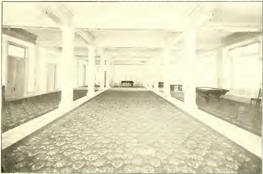
Grand Lobby, Hotel Victory.
