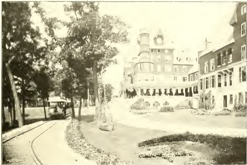
Main Entrance Hotel Victory, showing Victory Park Railway Terminal.
