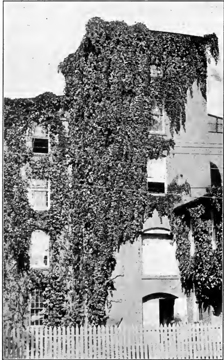
FIG. 156. A FACTORY COVERED WITH WOODBINE
