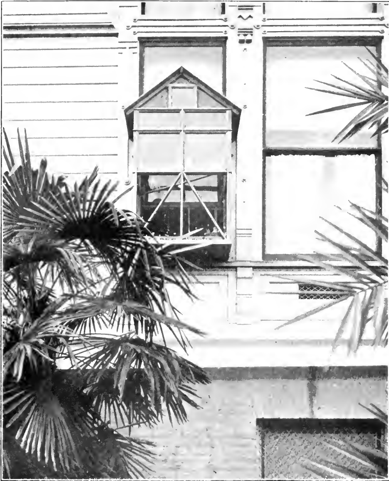
Window cage as seen from outside the building.
