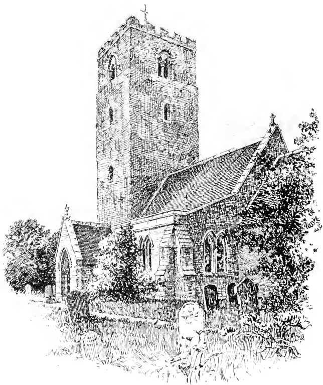
FIG. 176, Tower of Clapham Church, near Bedford.
