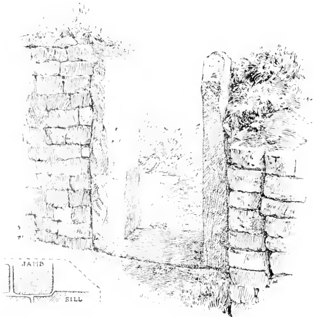
FIG. 26, Roman doorway at Chesters on the North Tyne, showing the monolithic jambs mortised into the sill and lintel.
