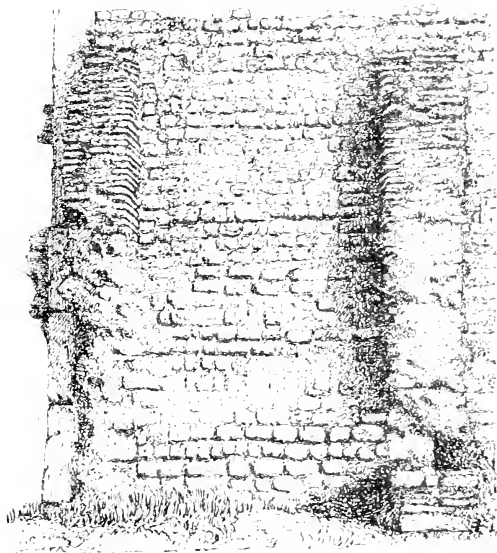
FIG. 48, Part of S wall of St Peter, Bradwell, Essex.
