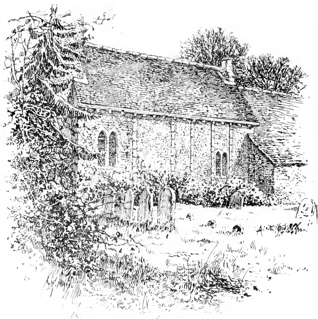
FIG. 7, Pilaster strips on the nave wall of Woolbeding Church, Sussex. The strips are about 7 in. in width.
