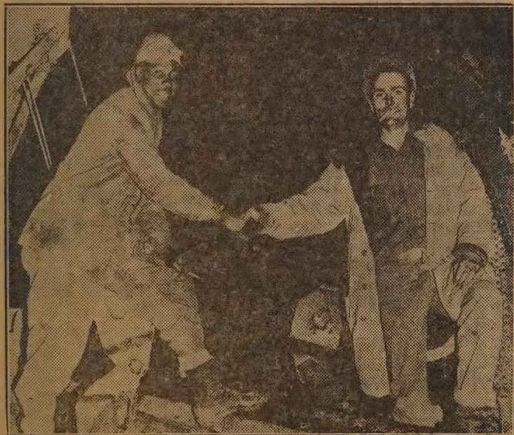
FINAL BREAK-THROUGH ON ALCAN HIGHWAY —Corporal Refines Sims, Jr., of Philadelphia, Pa., (left) and Private Alfred Jalufka of Kennedy, Texas, shake hands where their bulldozers met.
