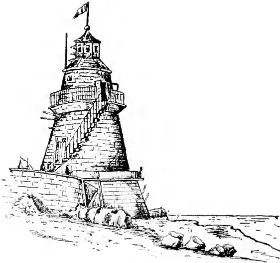
The Poolbeg Lighthouse in its original form.
