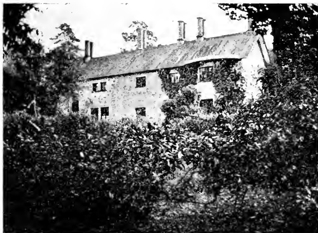
Glennasmole Lodge, formerly Heathfield Lodge. (1905.)
