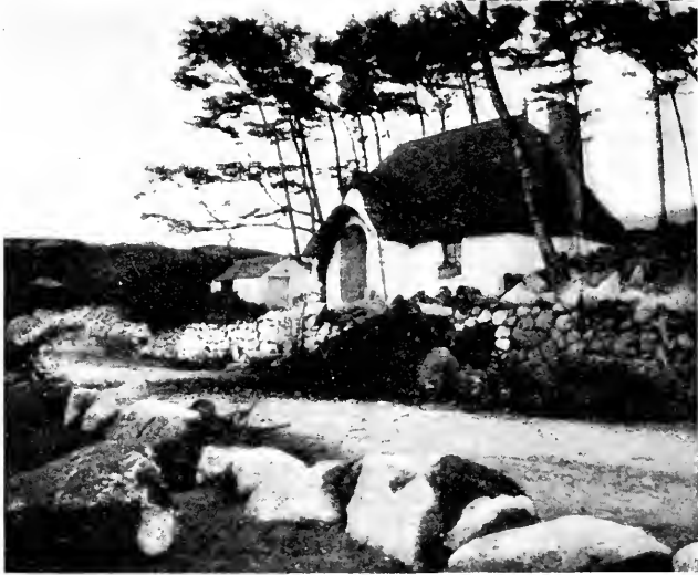
Cottage at Lough Bray. (1905.)
