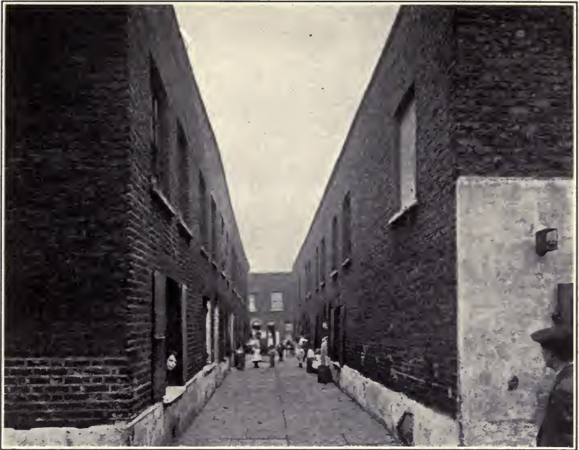
Tabard Garden Area. View, before clearance, of Boss Court
