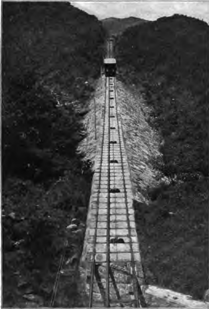
WIRE-ROPE TRAMWAY, HONG-KONG.
