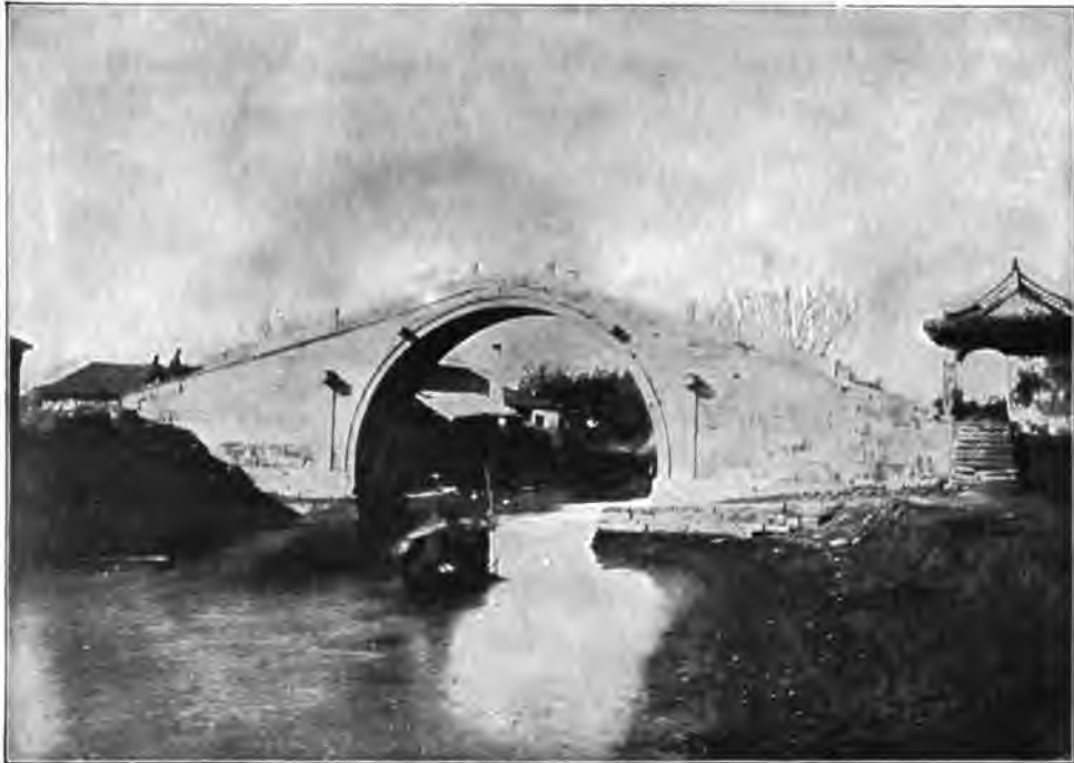
BRIDGE OVER CREEK AT KIASHAN.
