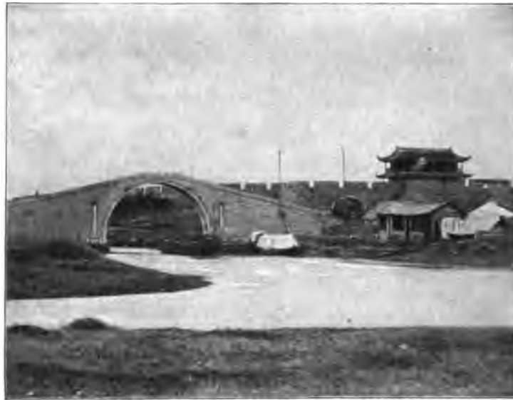
BRIDGE OVER CANAL AT SARCHOW.
