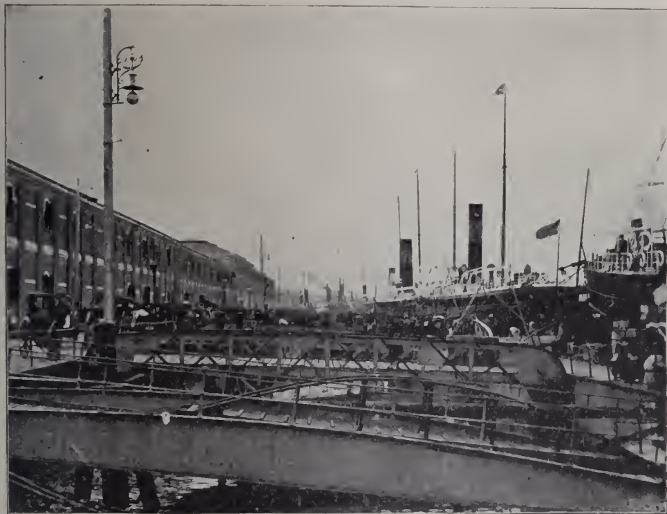
WHARF AND STOREHOUSES, SHANGHAI.
