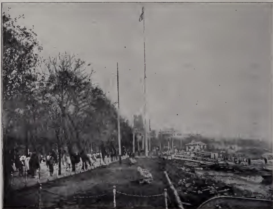
ROAD BY THE SIDE OF WANGPOO RIVER, SHANGHAI.
