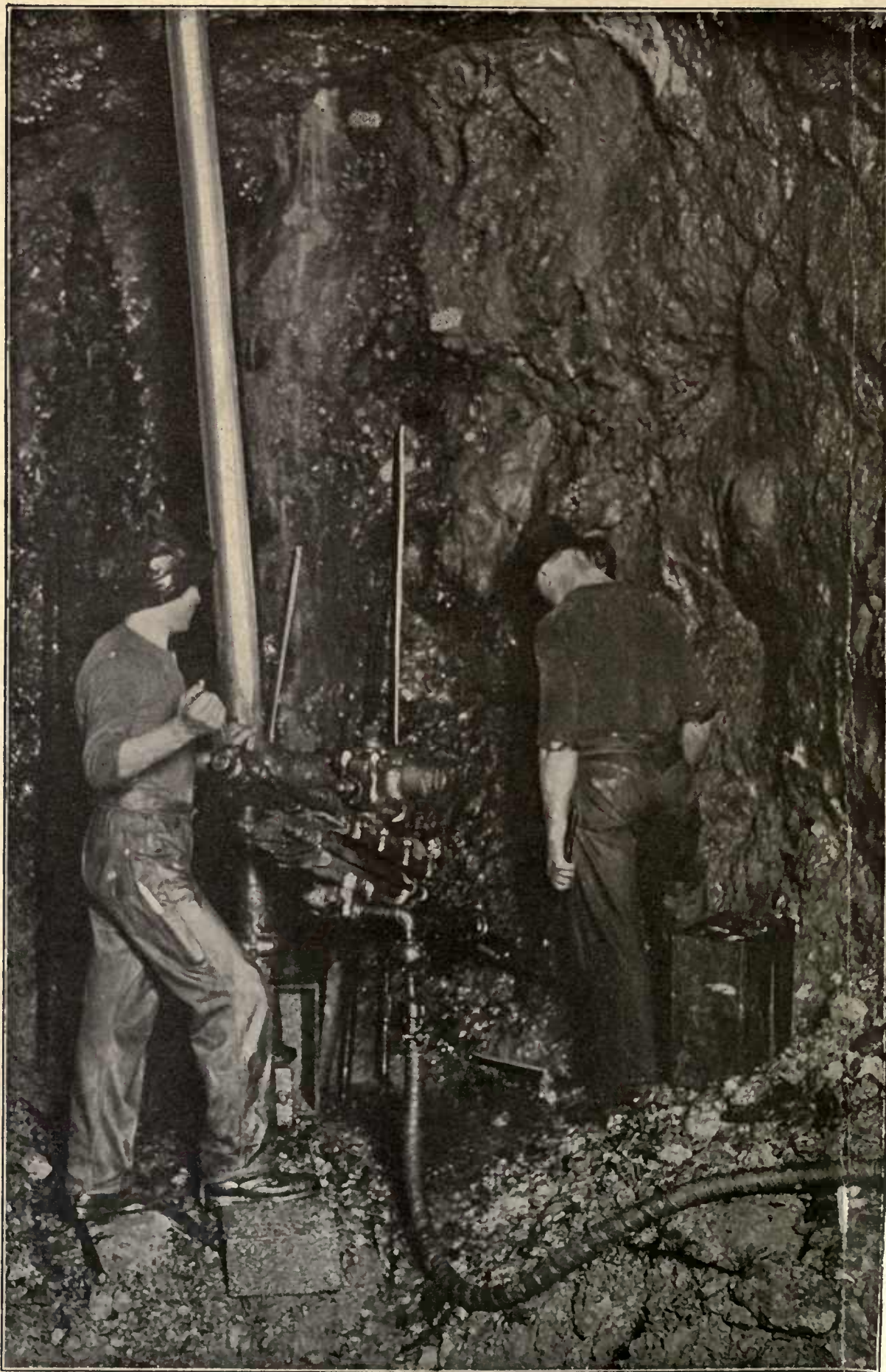
Compressed air drill in operation in one of Anaconda's mines. This shows the fundamental operation in mining—the starting-point of the Company's vast business. All of the wealth which Anaconda has produced has had its origin in the ore drilled and blasted as shown here.
