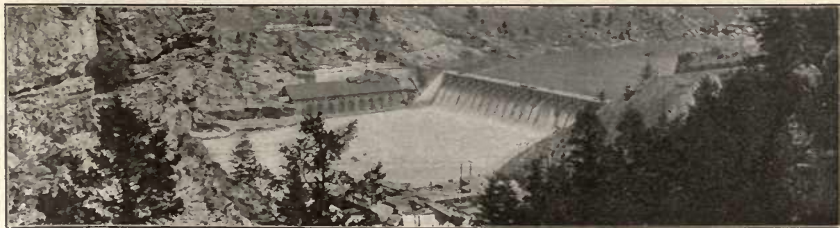
ONE OF ANACONDA'S IMPORTANT SOURCES OF POWER The Montana Power Company's Hydro-Electric Station at Hauser Lake.
