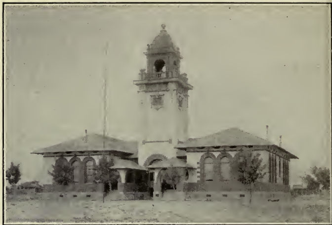
School Building, Tucson
