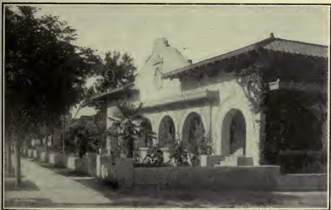
A Tucson Residence
