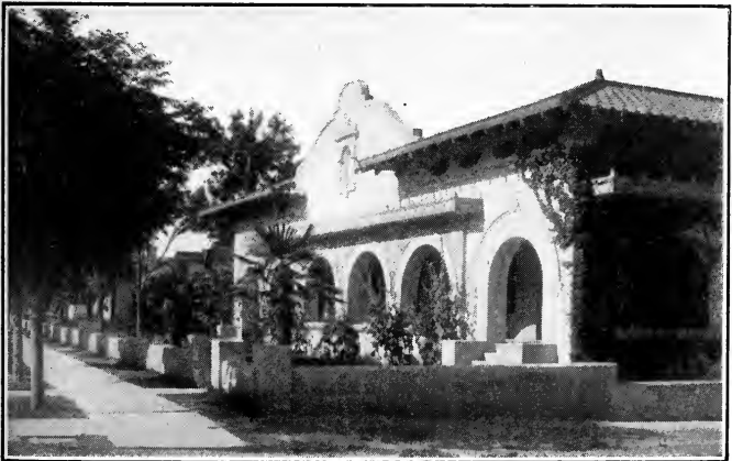
A Tucson Residence
