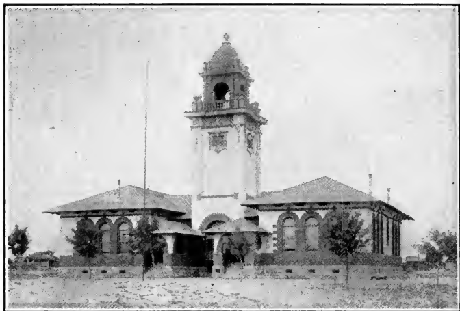
School Building, Tucson
