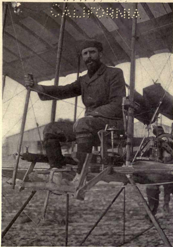
Fig. 28.—Henry Farman seated in his biplane. His hand grasps the lever by which the ailerons are operated
