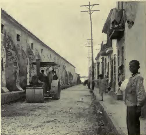
FACTORIA STREET, UNDER REPAIR
