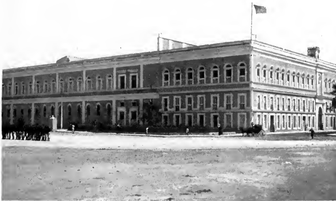
THE PRESENT POST-OFFICE BUILDING
