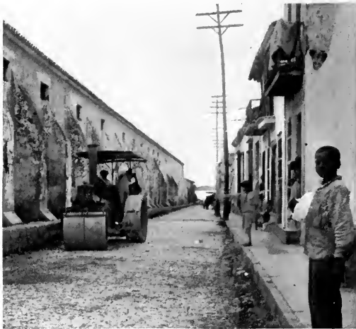
FACTORIA STREET, UNDER REPAIR
