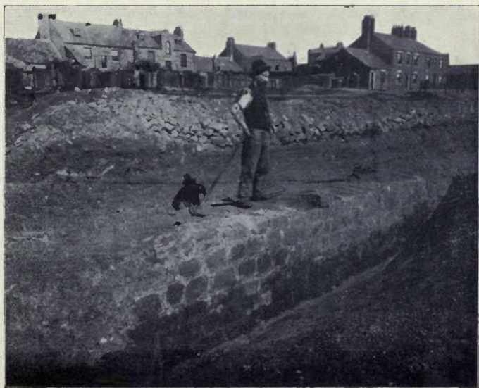
PORTION OF THE INSIDE OF THE EAST RAMPART
