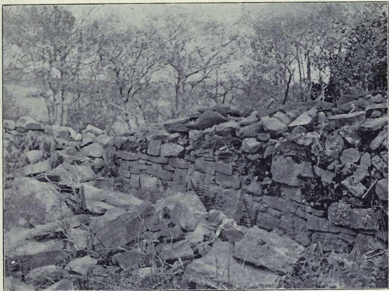
NO. 1, FROM THE INSIDE.
