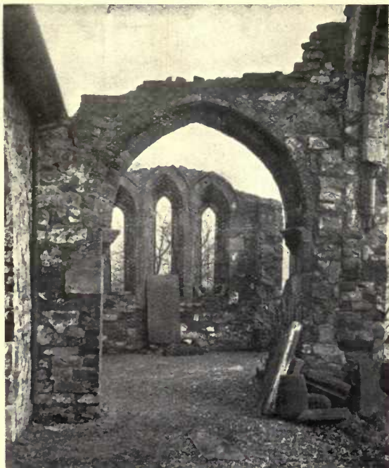
EAST END AND CHANCEL ARCH FROM INSIDE.
