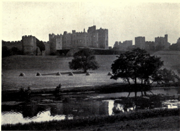
GENERAL VIEW FROM THE NORTH.
