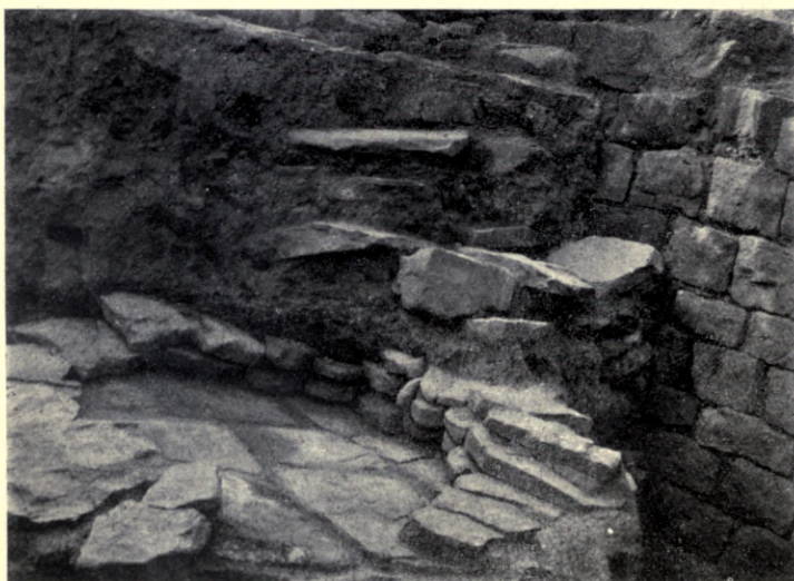
THE 'OVEN,' NORTH-WEST CORNER.
