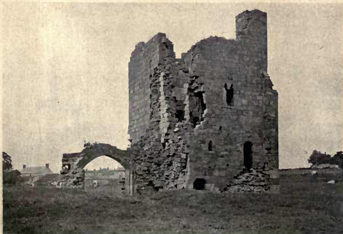
GATEWAY TOWER, RAVENSWORTH CASTLE, N. YORKS
