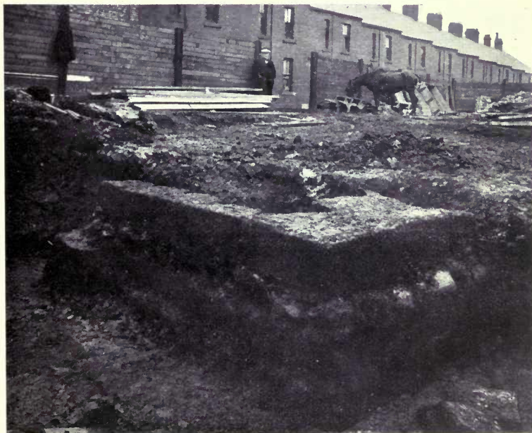
FOUNDATION OF NORTHERN GUARD CHAMBER, EASTERN GATEWAY.
