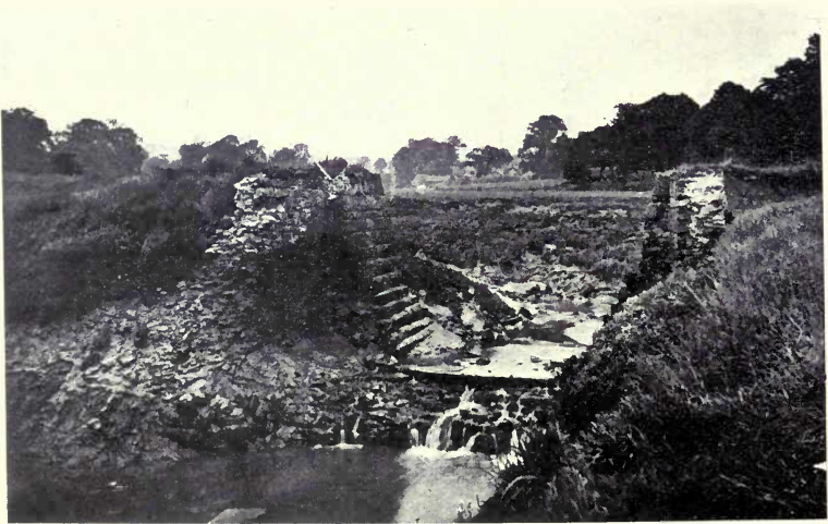
UPPER GATEWAY LOOKING UP STREAM. The sill of the gate arches down stream; it is paved between piers. Remains of timber in square recess at each corner.
