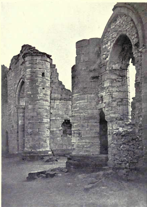
S.W. AND N.W. PIERS OF CROSSING FROM NORTH TRANSEPT.
