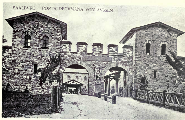
RESTORATION OF DECUMAN GATE (FROM OUTSIDE).
