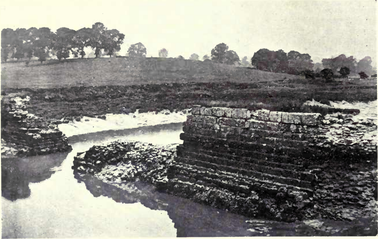
DOWNSTREAM GATEWAY. Wall-casing mostly gone leaving rubble core.
