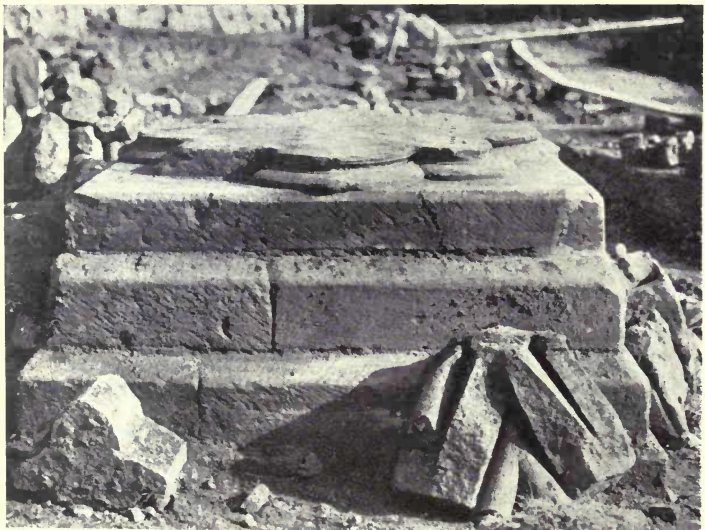
PLINTH OF COLUMN IN SOUTH TRANSEPT.
