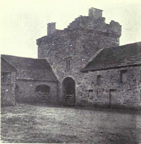
WILLIMOTESWICK CASTLE: GATE TOWER FROM THE INSIDE.
