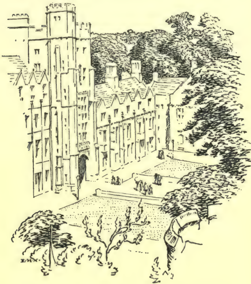
HOLYWELL BUILDINGS AND ROBINSON TOWER FROM THE CHAPEL ROOF
