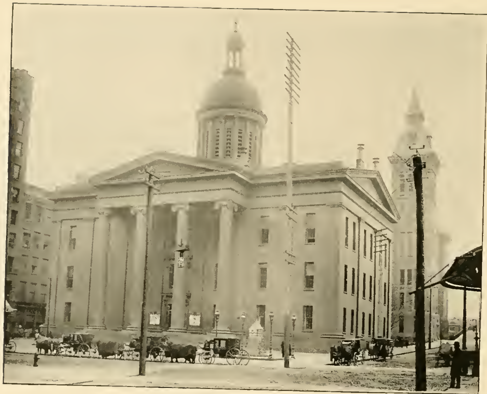
SECOND MONROE COUNTY COURT HOUSE.
