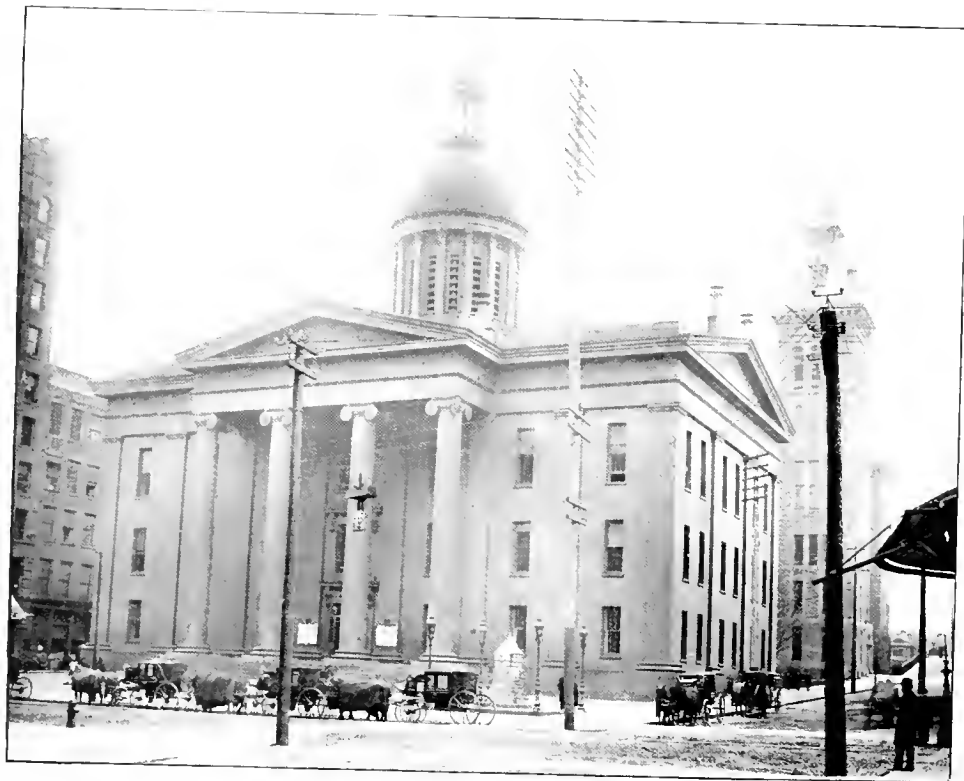
SECOND MONROE COUNTY COURT HOUSE.
