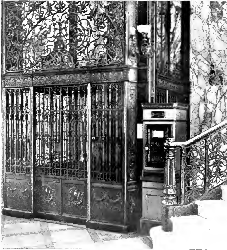
U. S. MAIL CHUTE AND BOX IN MAIN CORRIDOR.
