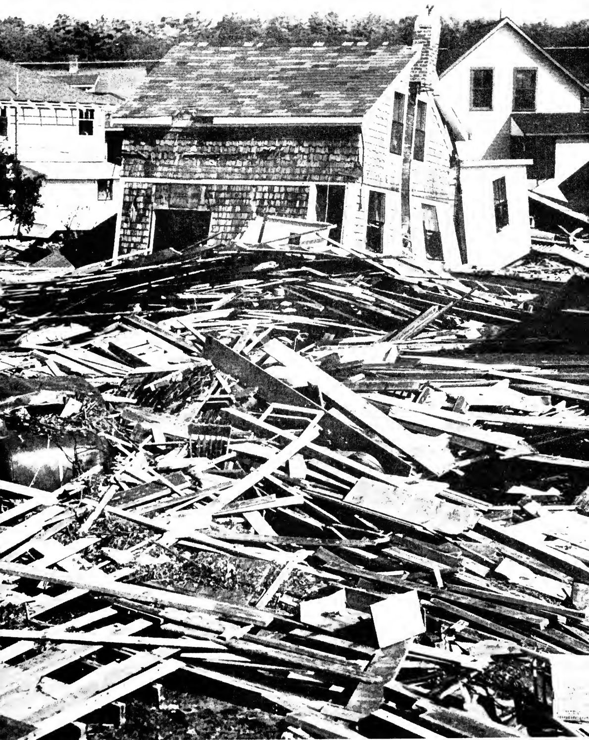
Nine lives were lost and 300 houses totally destroyed by the wind-flung tide which drove high up on the shores of MATTAPOISETT. The beaches were buffeted, none more so than Crescent Beach where all but 10 of the 170 cottages were ruined. The automobile nearly buried in the left center of the photograph shows the accumulation of wreckage.
