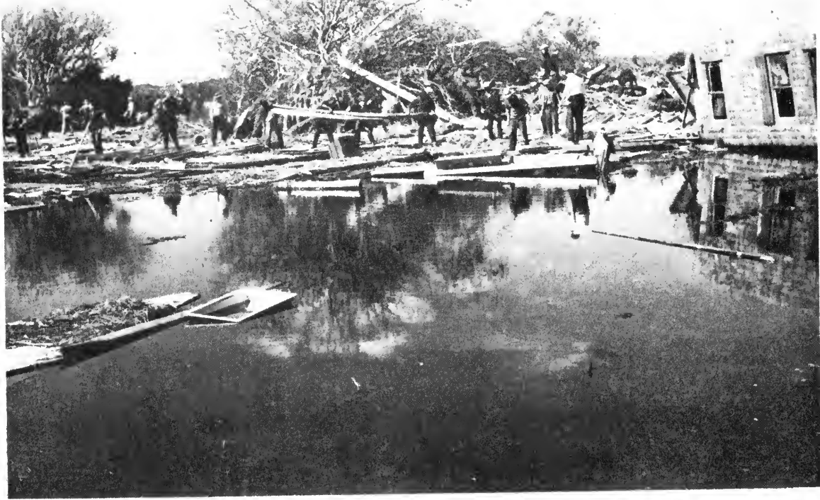
The first efforts of WPA workers were directed towards finding the corpses of Charlestown victims. Refuse pushed aside by searchers was piled up for later burning.
