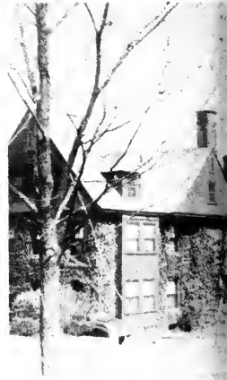
On Salisbury the Central C roof was hach
