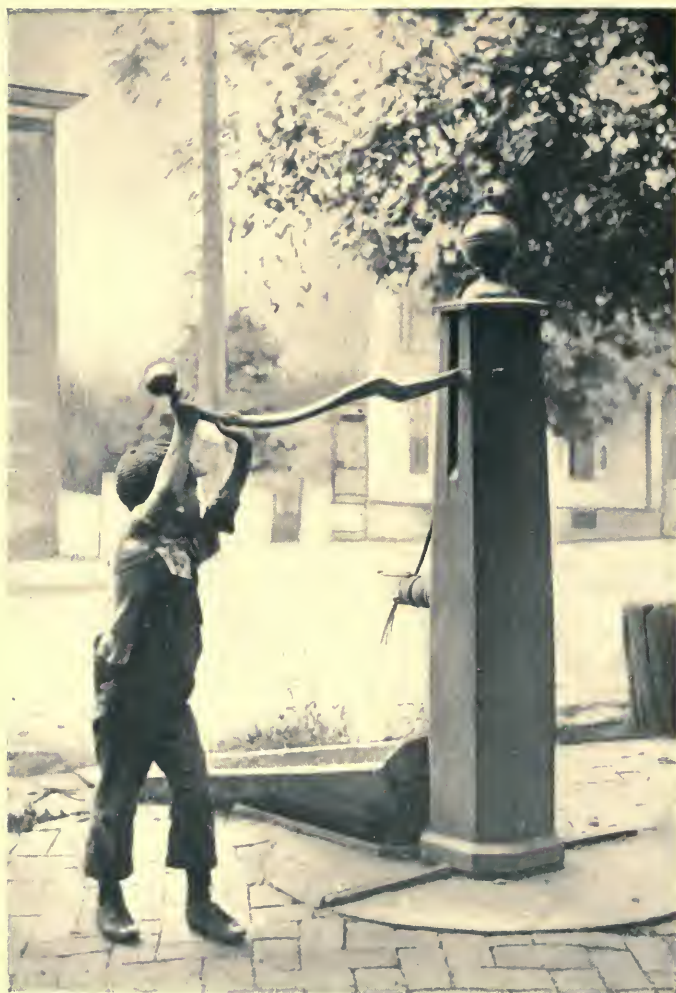
ONE OF THE STREET PUMPS
