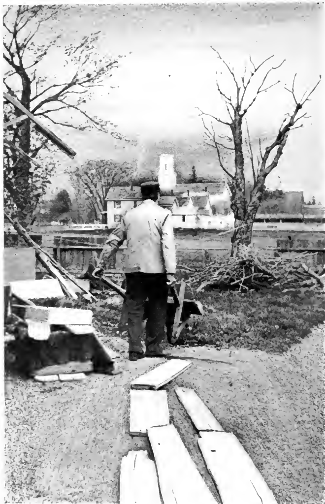
CLEANING UP THE BACK YARD
