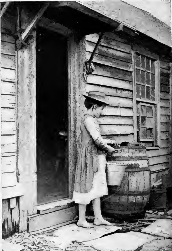
The Rain-water Barrel
