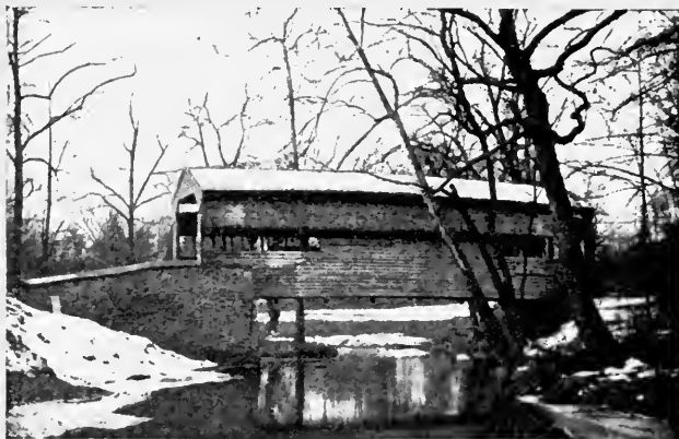
One of the Bridges over "Valley Crick"
