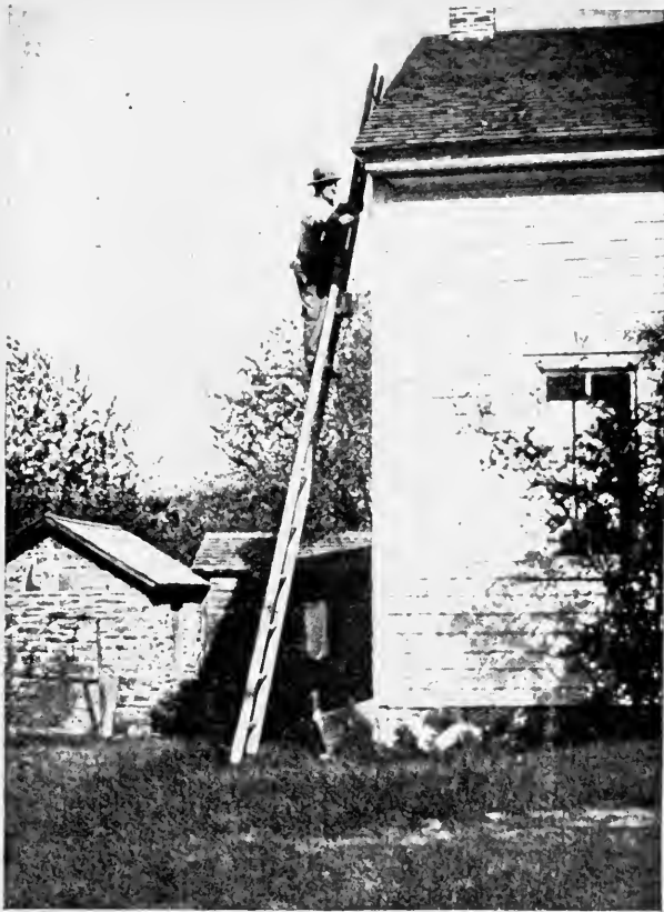
Putting on a Fresh Coat of Paint
