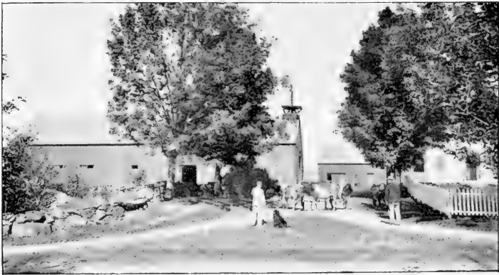
FARM BUILDINGS OF H. F. CATER, BARRINGTON.
