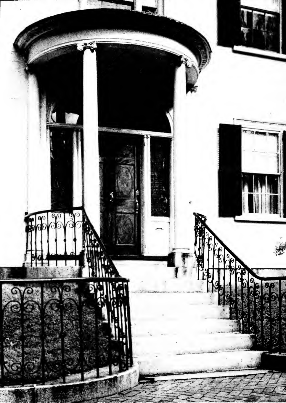
PORCH, LANGLEY BOARDMAN HOUSE, PORTSMOUTH
