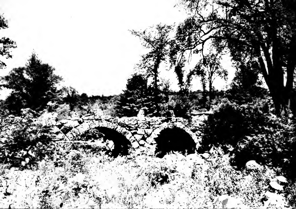
OLD STONE BRIDGE, HILLSBOROUGH
