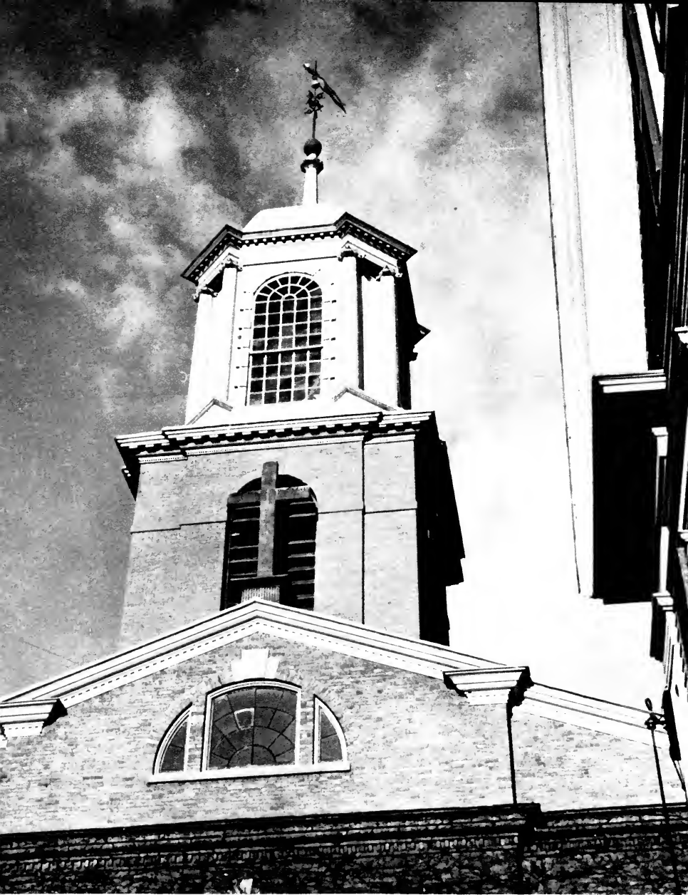
ST. JOHN'S CHURCH TOWER, PORTSMOUTH
