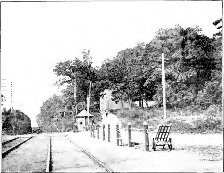
INWOOD STATION, ON THE N. Y. CENTRAL R. R.
