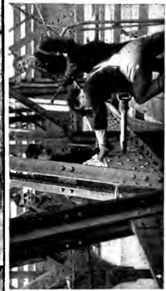
1. EXPANDING BOILER TUBES
