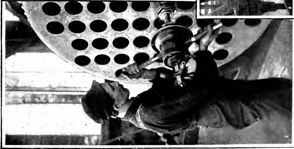
1. EXPANDING BOILER TUBES
