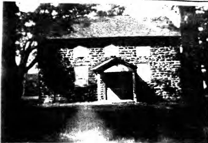
Figure 81 Arny's Mount Meeting House, main facade, T. Chalkey Matlack Collection Historical Society Of Pennsylvania
