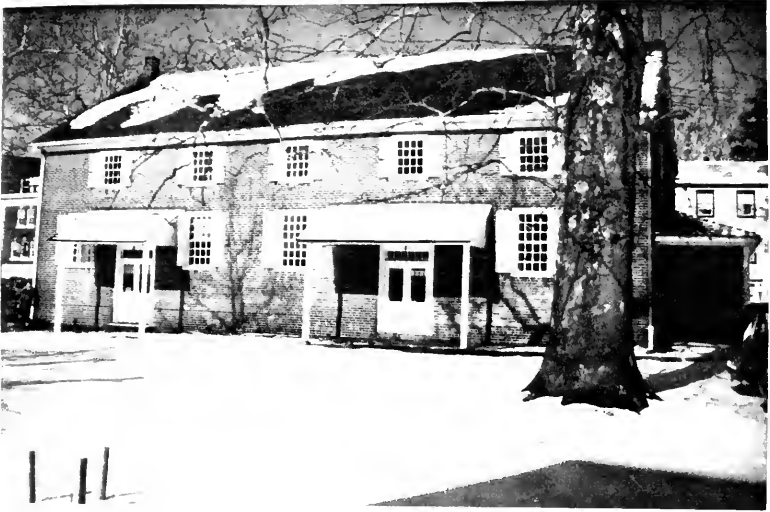
Figure 105 Mount Holly Meeting House main facade author's photo
