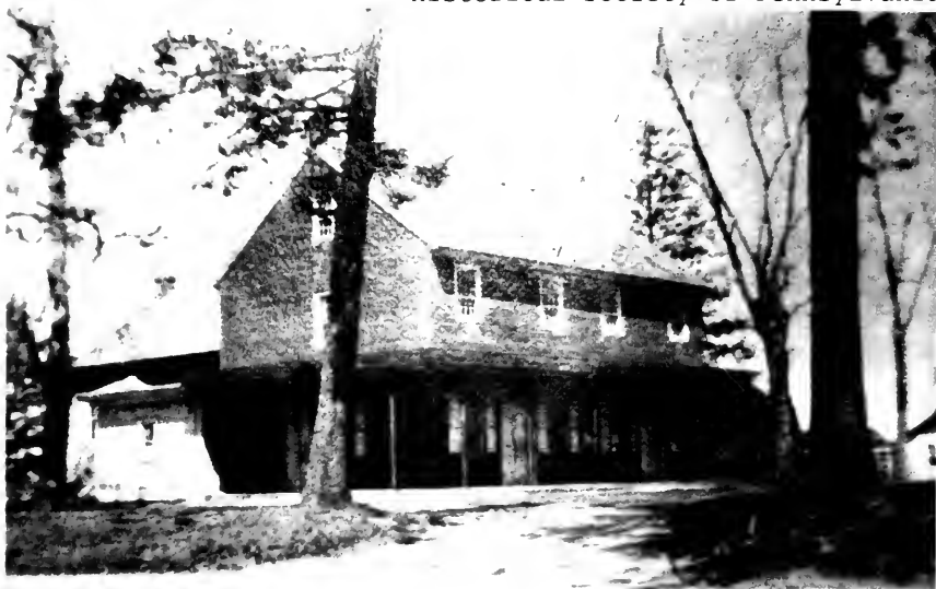
Figure 191 Upper Greenwich Meeting House T. Chalkey Matlack Collection Historical Society of Pennsylvania
