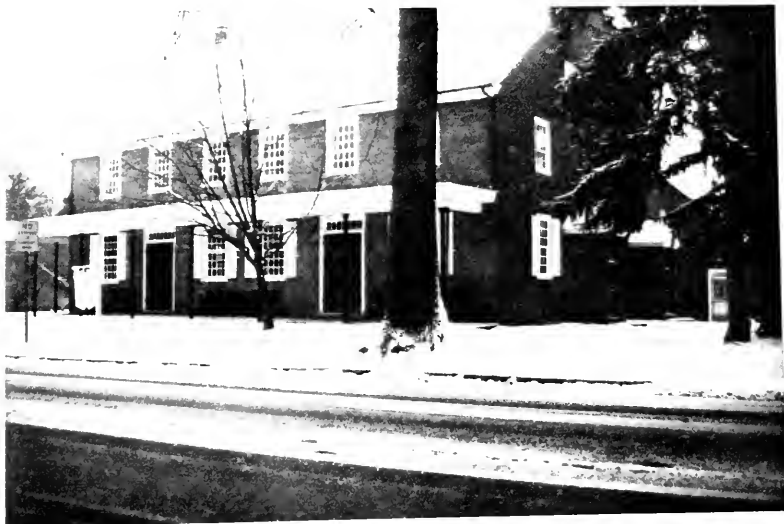
Fig. 46 Pilesgrove Meeting House Author's Photo
