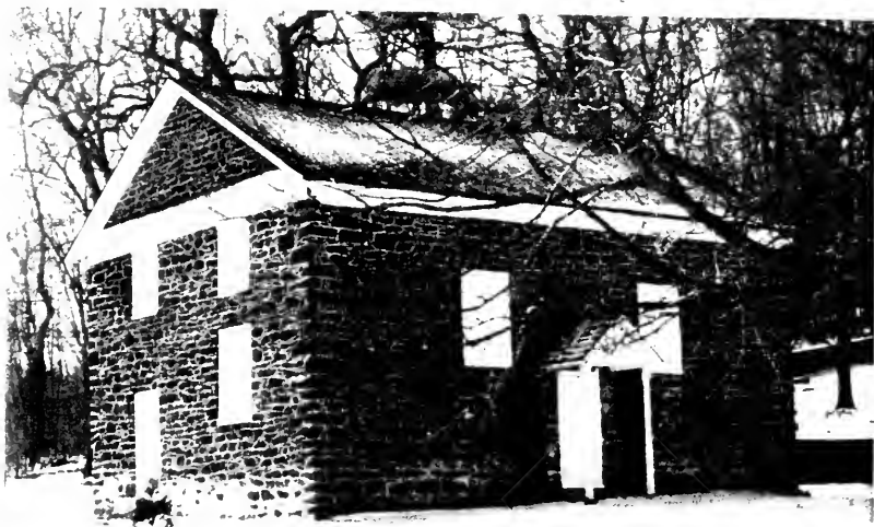
Figure 82 Arny's Mount Meeting House street facade, author's photo
