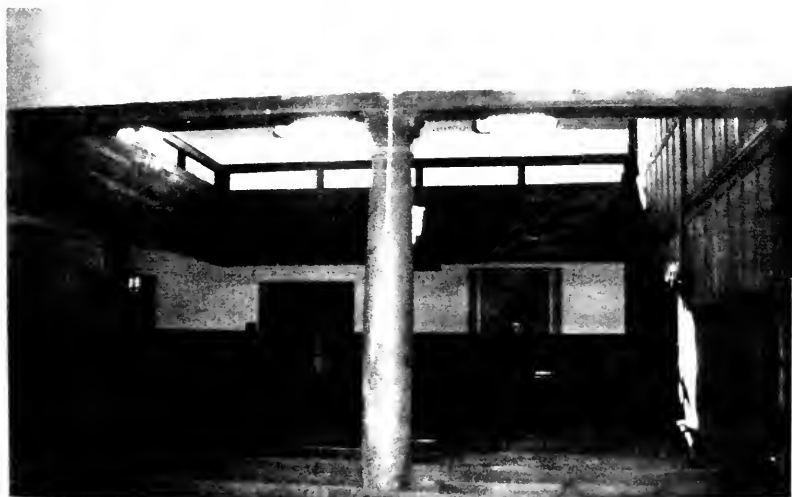
Figure 92 interior, Burlington Meeting House author's photo
