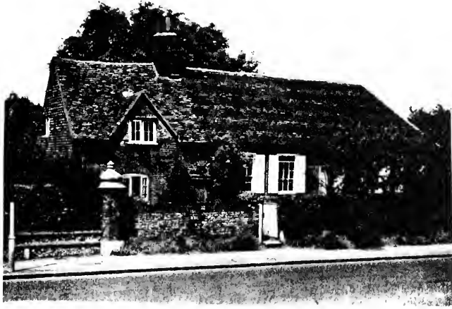
Fig. 5a, Photo Amersham Meeting House. Taken from Hubert Lidbetter, The Friends Meeting House .
