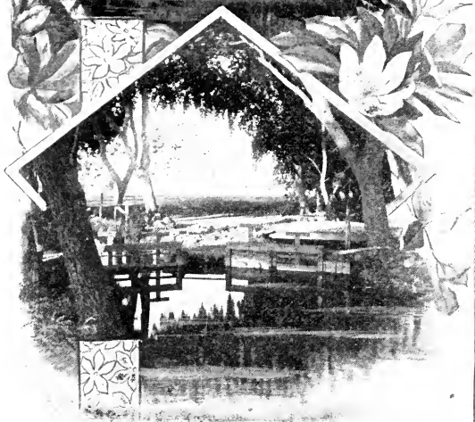
PECOS RIVER FLUME. THE CHISUM DITCH. DIVIDING WATER AT CHISUM RANCH.
