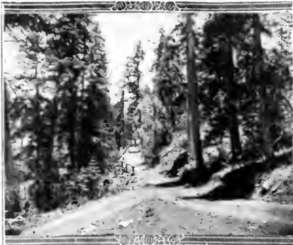
TYPE OF ROAD CONSTRUCTED BY THE FOREST SERVICE
