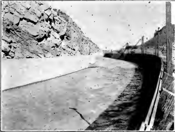
THE BIG FLUMES (NOW CLOSED) BY WHICH THE RIO GRANDE WAS CONDUCTED PAST THE DAM WHILE THE LATTER WAS BEING BUILT
