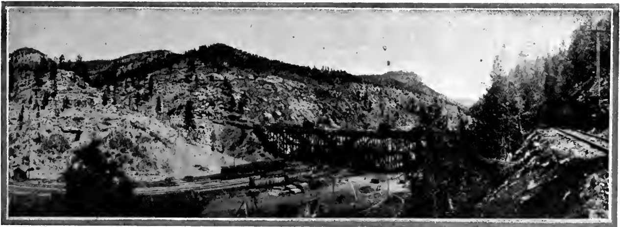
VIEW OF TIPPLE—SHOWING SHIPPING FACILITIES AT KOEHLER MINE
