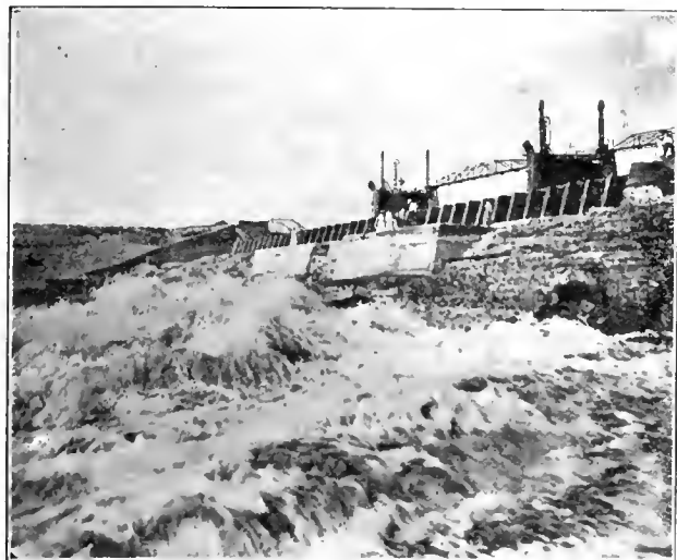
TUNNEL SPILLWAY-OUTLET—CARLSBAD PROJECT—LAKE AVALON
