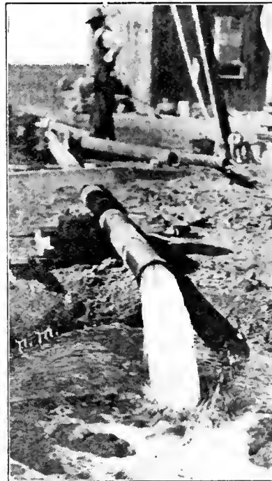
PUMPING NEAR TULAROSA
