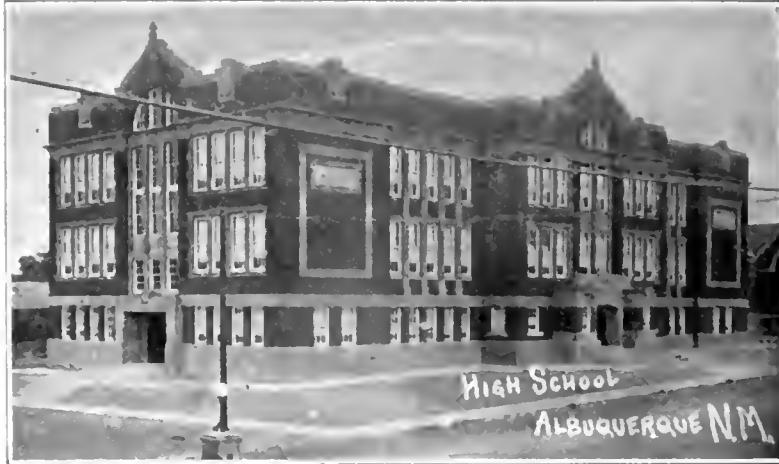
ALBUQUERQUE'S NEW HIGH SCHOOL BUILDING, LYON & AXTELL CO., BUILDERS
