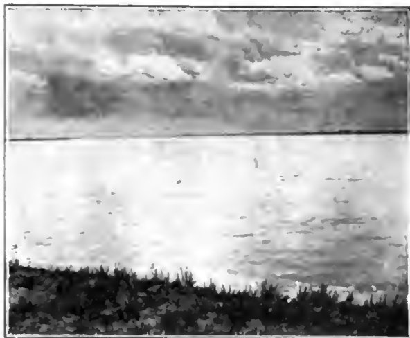
ONE OF THE RESERVOIRS ON MAXWELL PROJECT
