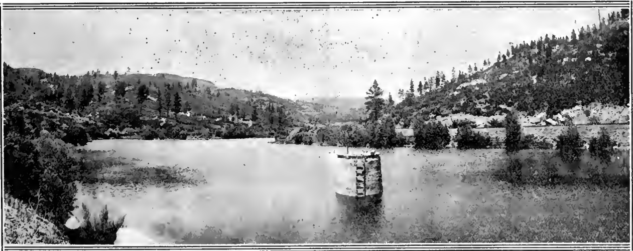
ONE OF NEW MEXICO'S MANY BEAUTIFUL WATER SUPPLY LAKES
