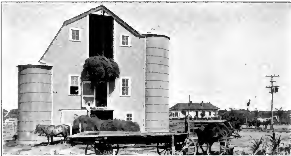
ELECTRIC DAIRY BARN—ROSWELL
