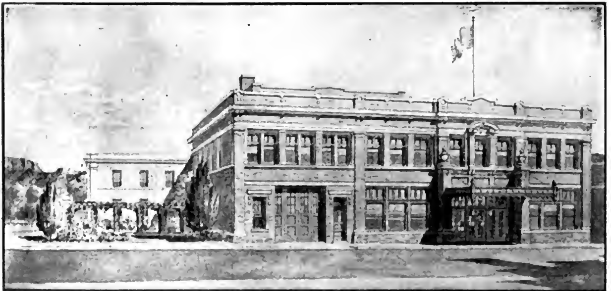
RATON'S HANDSOME AND COMMODIOUS CITY HALL AND MUNICIPAL BUILDING
