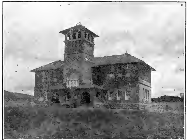
CIMARRON SCHOOL BUILDING
