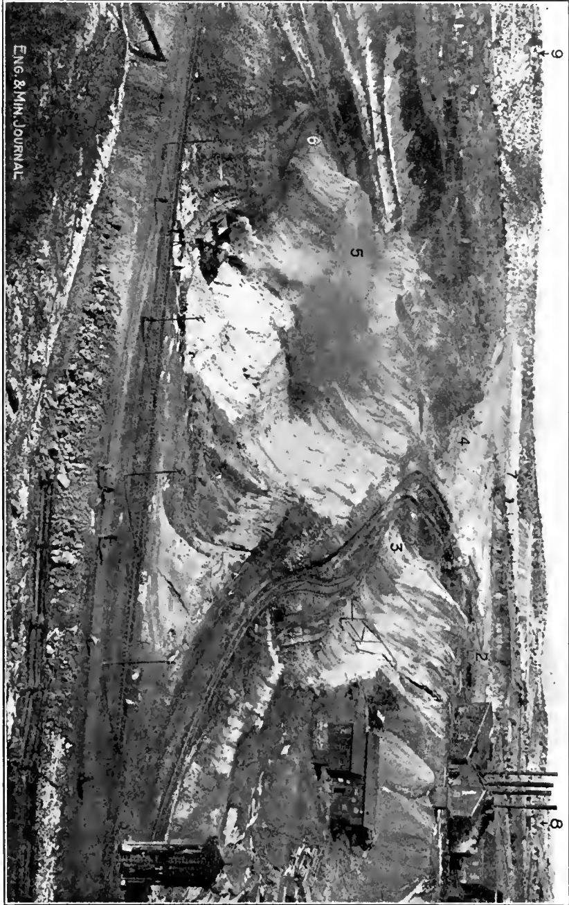
VIEW FROM EAST HILL, LOOKING WEST THROUGH NORTHEAST OREBODY PIT FROM EAST SIDE OF WORKS 1. Santa Rita Hoist House. 2. 6370 Bench. 3. 6310 Bench, Northeast Orebody. 4. 6300 Bench Connecting Northeast and West Orebodies. 5. 6280 Bench. 6. 6250 Bench, Northeast Orebody. 7. Waste Dump No. 3. 8. Booth Hill Company Houses. 9. Lee Hill.
