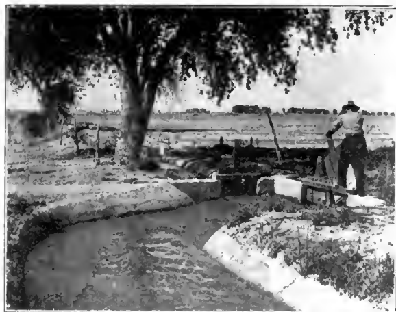
SYSTEM OF HEAD-GATES USED ON MAIN LATERALS—CARLSBAD PROJECT
