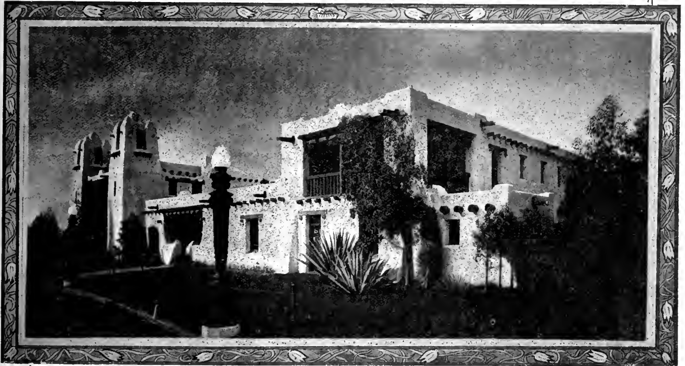
NEW MEXICO BUILDING — PANAMA-CALIFORNIA EXPOSITION
