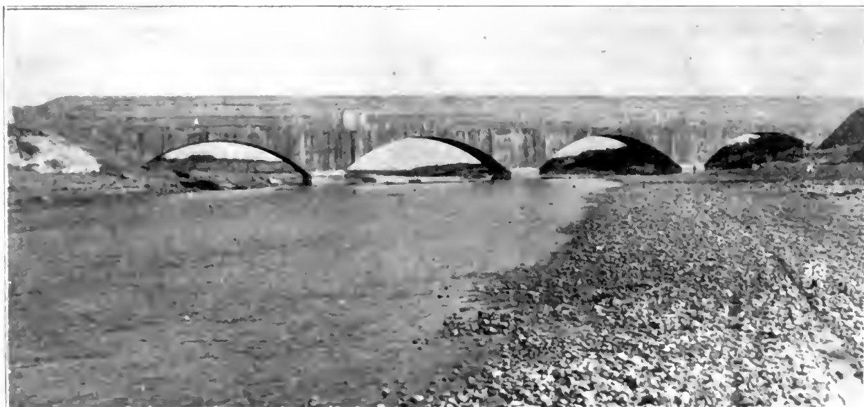
CONCRETE AQUEDUCT ACROSS PECOS RIVER—CARLSBAD PROJECT
