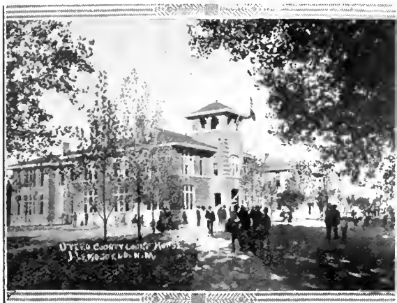
OTERO COUNTY COURT HOUSE AT ALAMOGORDO
