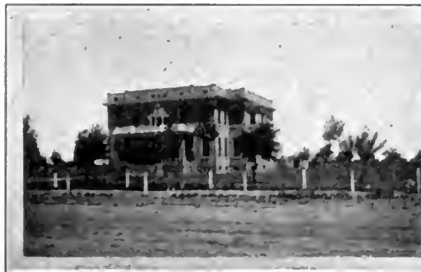
CURRY COUNTY COURT HOUSE AT CLOVIS
