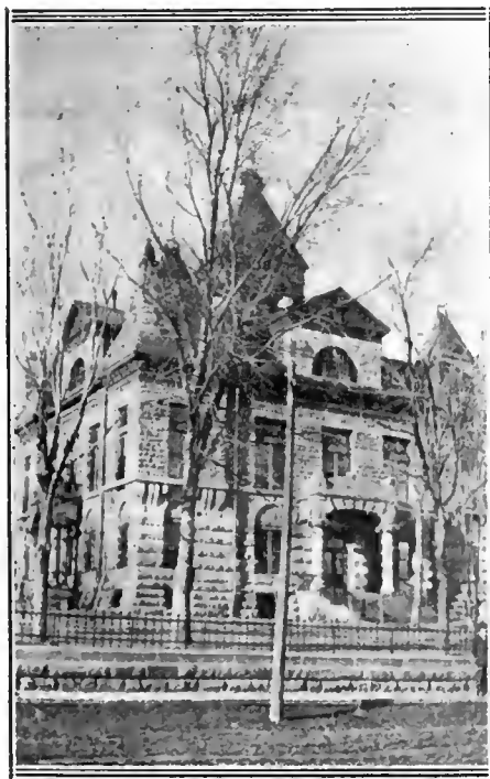
COUNTY COURT HOUSE, LAS VEGAS
