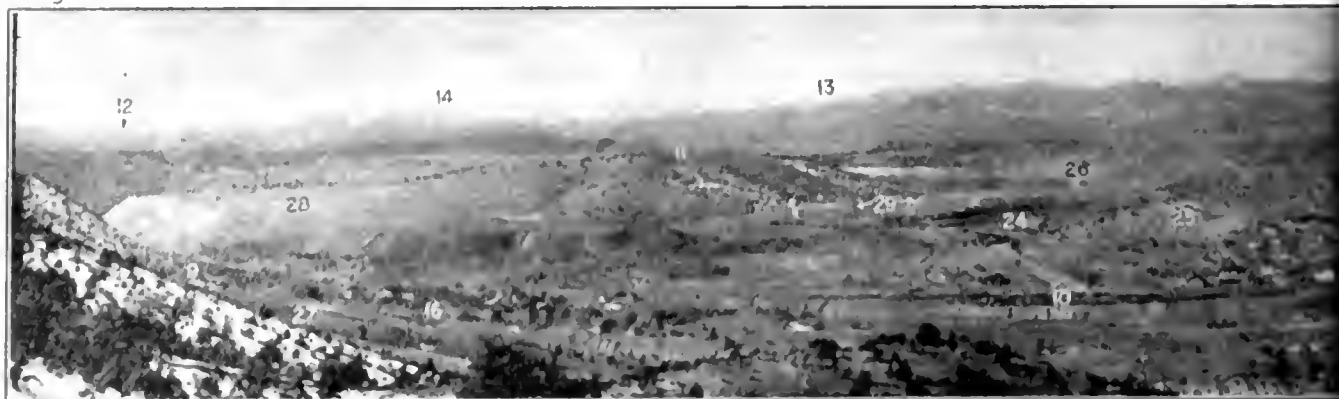
VIEW OF MINE WORKINGS 1. Booth Hill Company Houses. 2. Santa Rita Hill Company Houses. 3. Staff Houses. 4. Warehouse. 5. Machine Shop. 6. Santa Rita Hill. 12. Bear Mountain. 13. Twin Sisters. 14. Pinos Altos. 15. Divide Between Santa Rita and Danover Gulches. 16. Santa Rita Hill. 23. 6370 Bench, Northeast Orebody. 24. 6300 Bench, West Orebody. 25. Waste Dump No. 8
