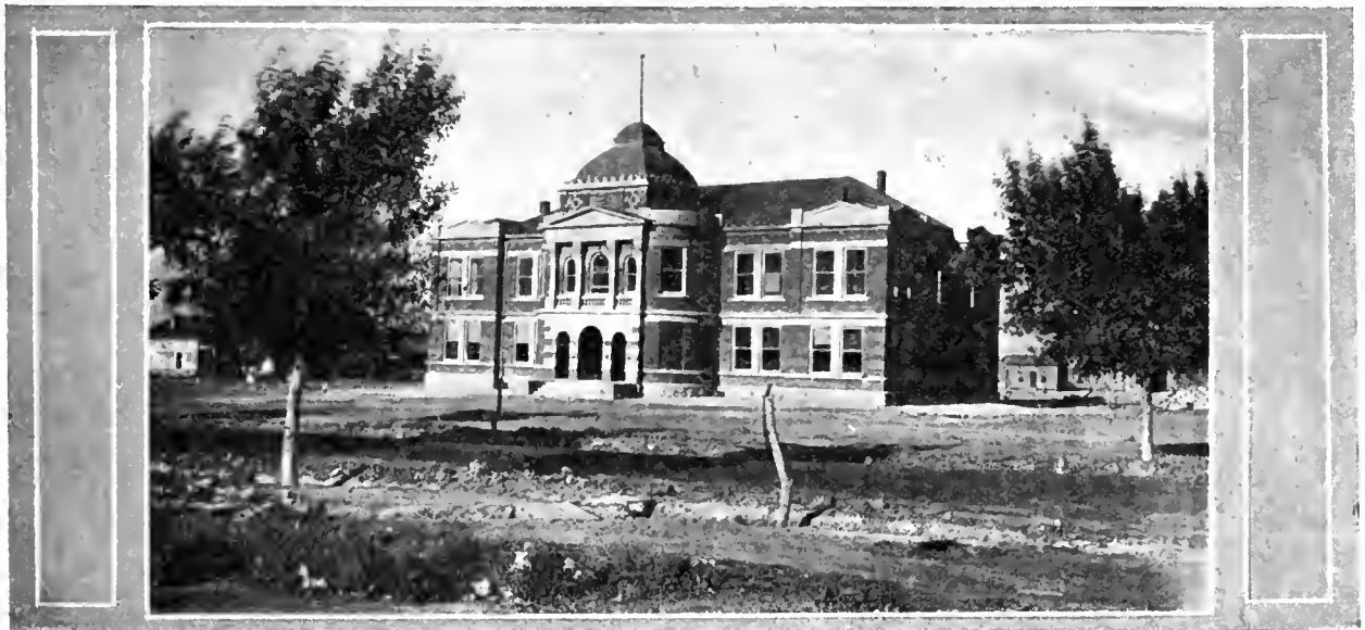
LINCOLN COUNTY COURT HOUSE AT CARRIZOZO
