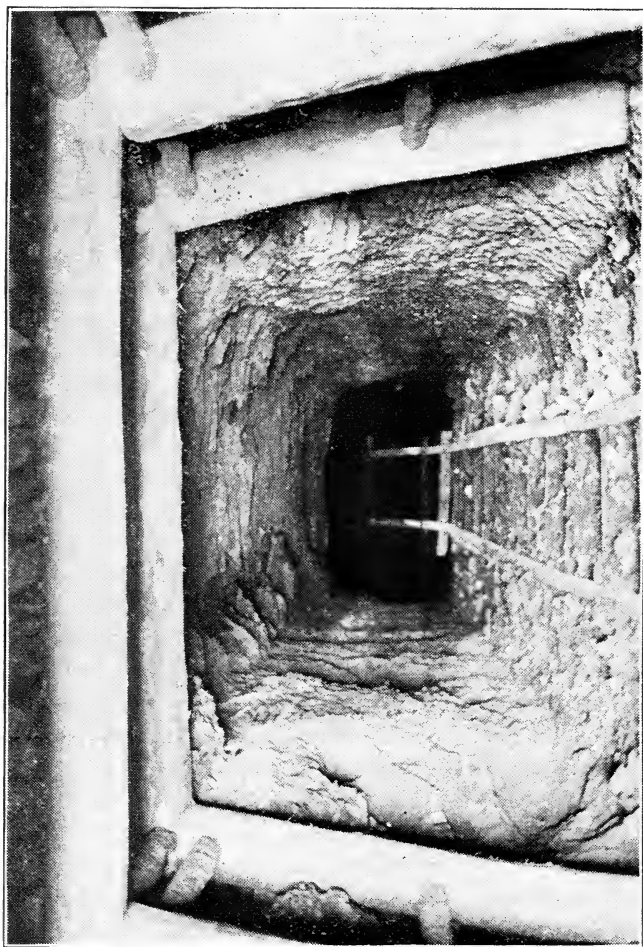
FIG. 37—OPENING AT THE PINAVITITOS COAL MINE.
