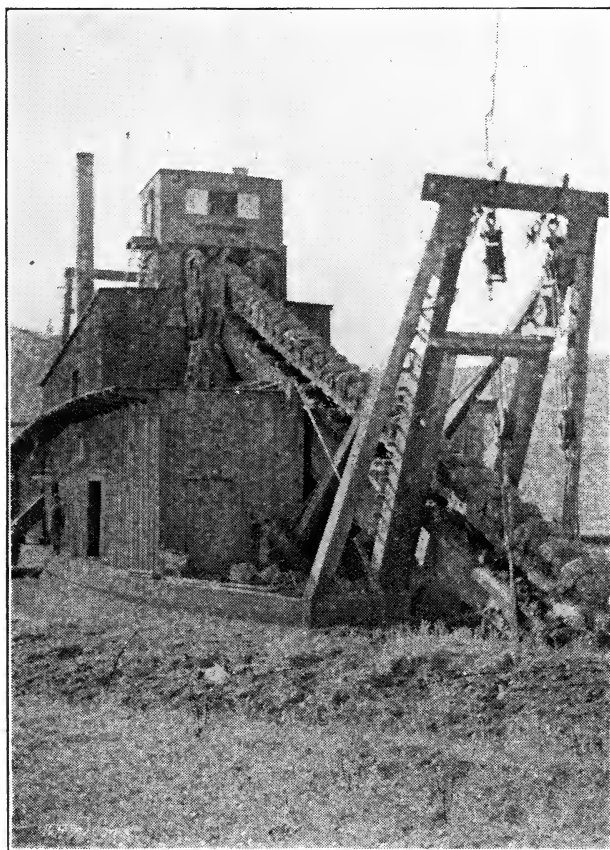
Fig. 27—DREDGE OF THE ORO DREDGING COMPANY, OPERATING IN THE MORENO RIVER AT ELIZABETHTOWN.
