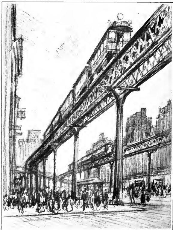
PL. 54. — ELEVATED ROAD ON THE BOWERY
