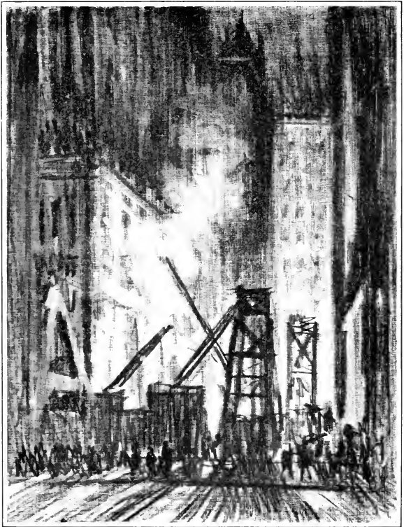
PL. 22. — WORKING AT NIGHT ON FOUNDATIONS
