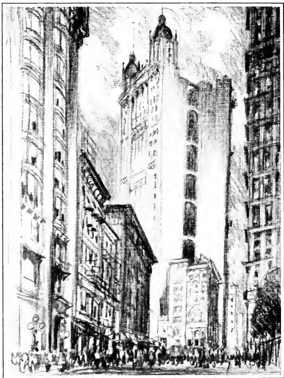
PL. 17. — PARK ROW BUILDING
