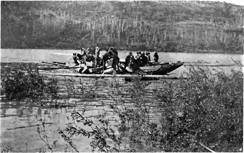
Towing the Wrecked Barge Ashore
