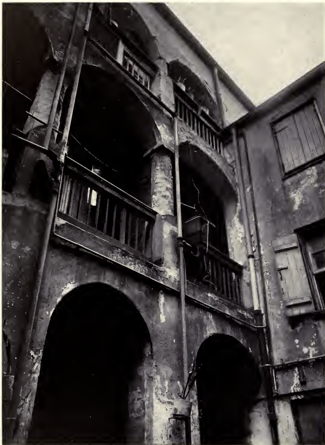
Back of Main Building from Courtyard
