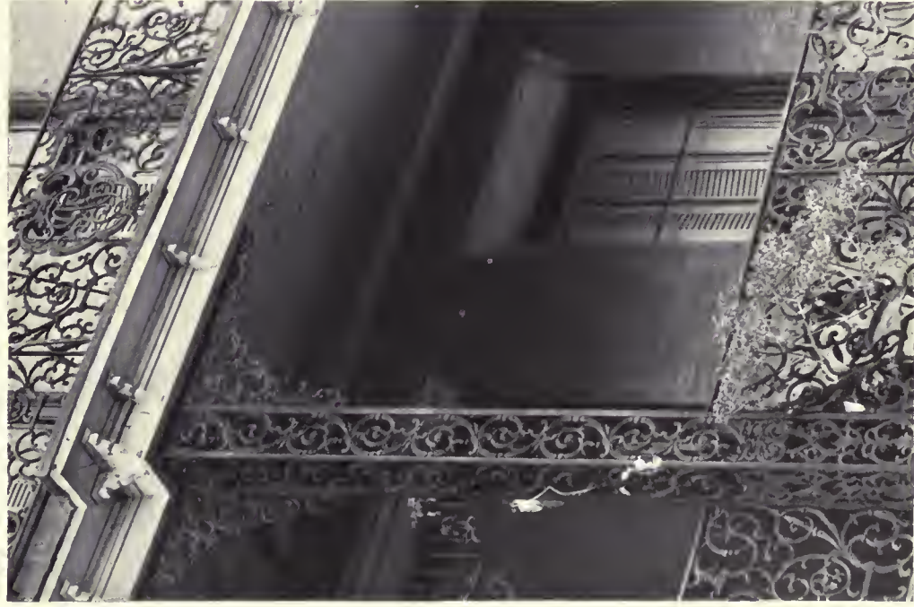
Cast Iron Balcony Details
