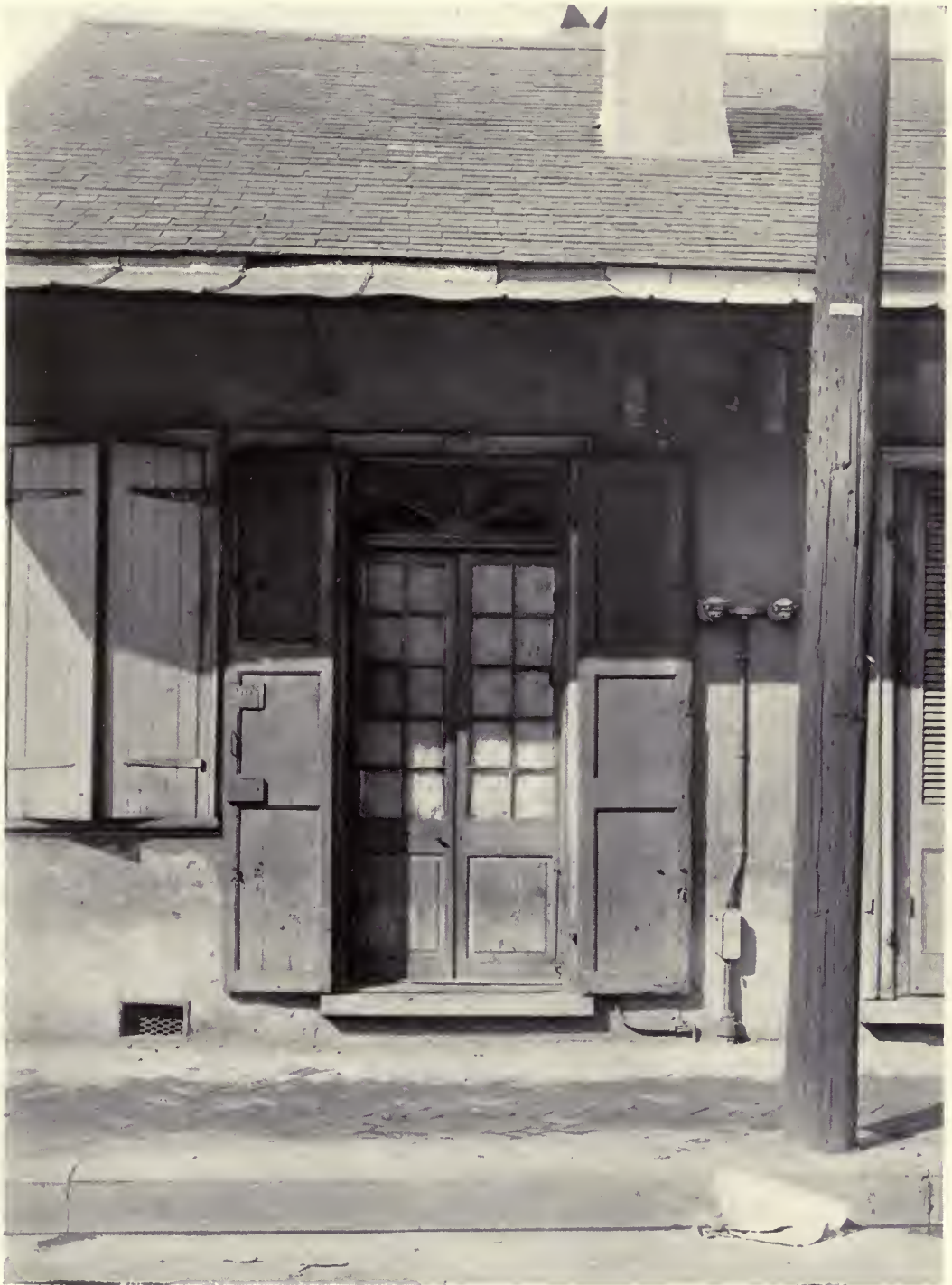
Entrance Door and Transom
