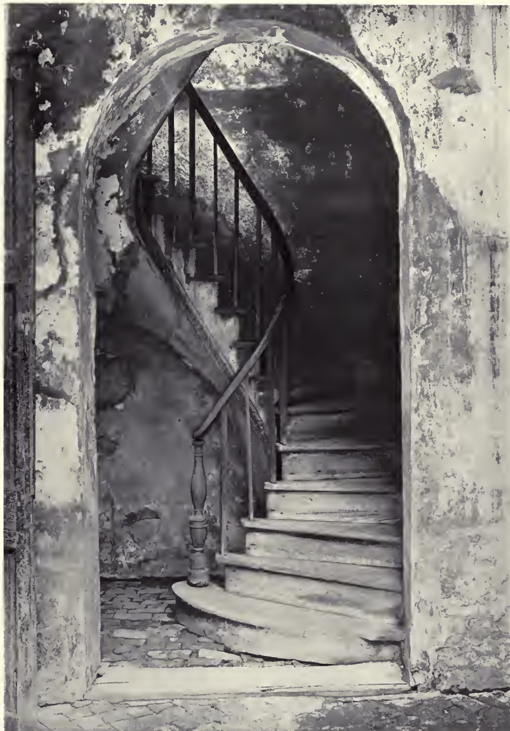
Courtyard Stair to Apartments Above House Illustrated, 8
