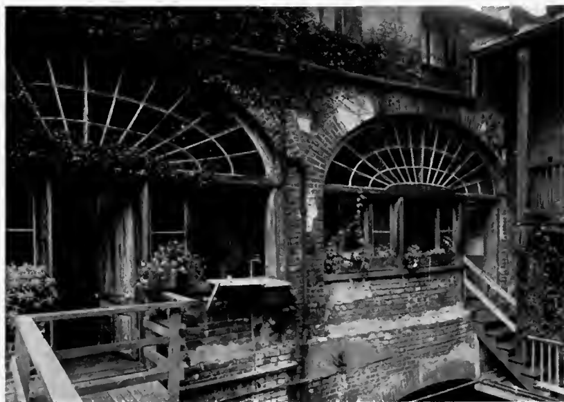
Fanlight Windows Overlooking Courtyard
