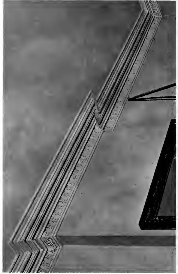
Plaster Cornice Detail
