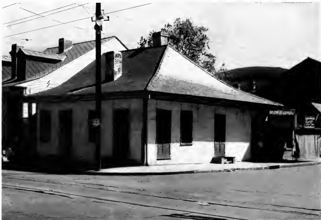
Note Double Pitched Roof and Large Overhanging Eaves DUMAINE STREET
