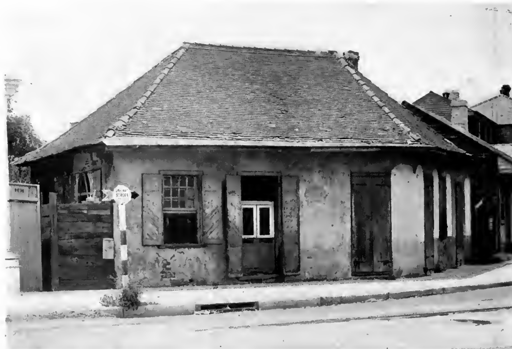
This Cottage Has One of the Few Remaining Flat Tiled Roofs Which, Shipped from Nantes, France, Were Used after the Fires of 1788 and 1794
