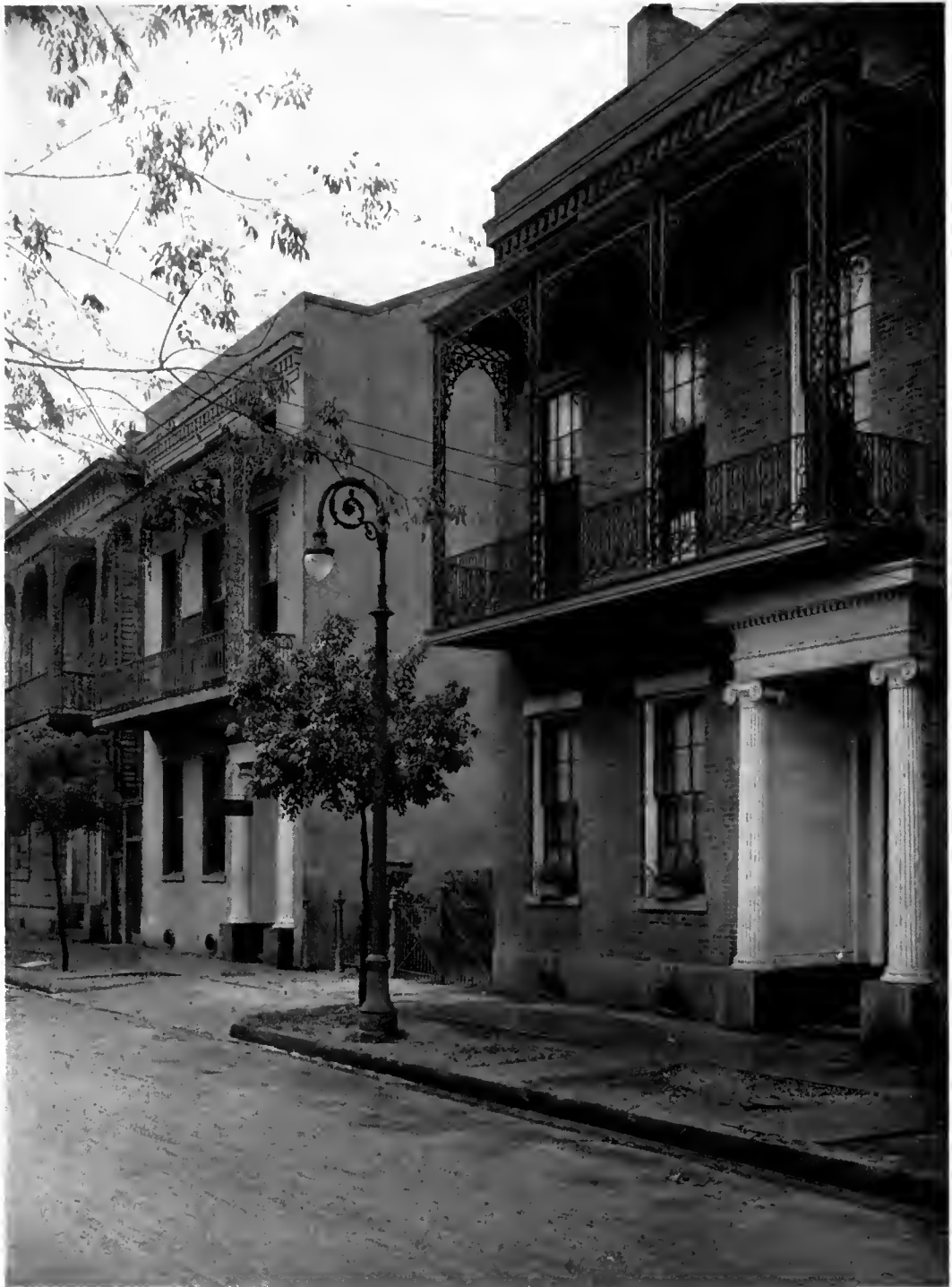
Typical Two and One-Half Story Buildings
