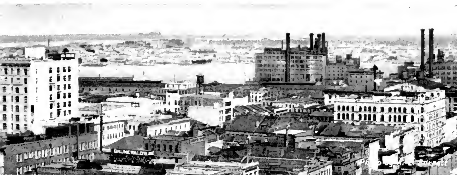
Viewing Crescent Bend
