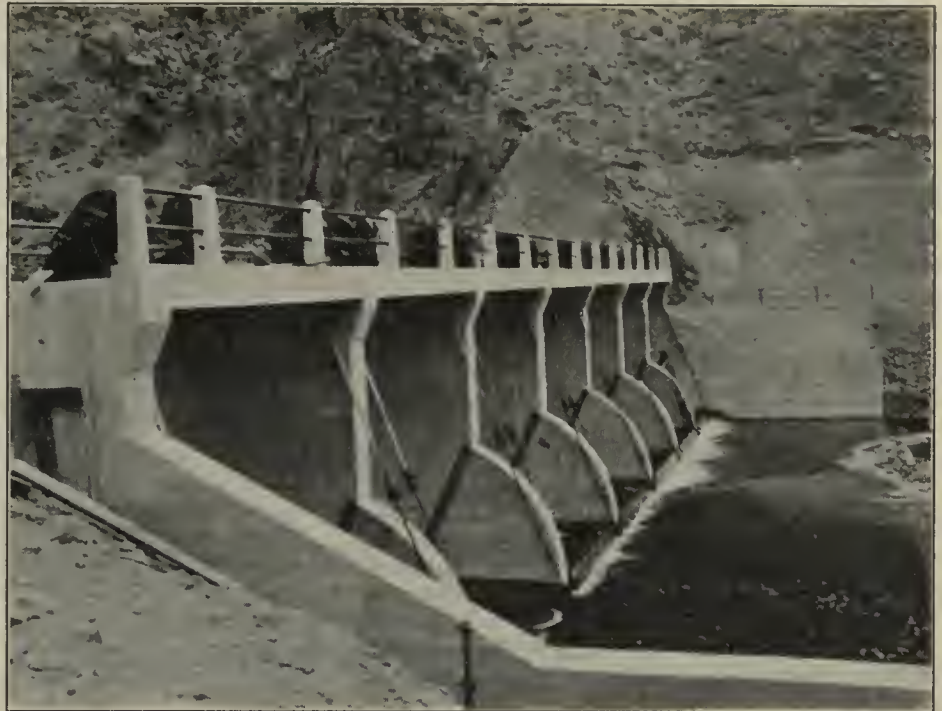
Harper diversion dam, Vale project, Oregon
