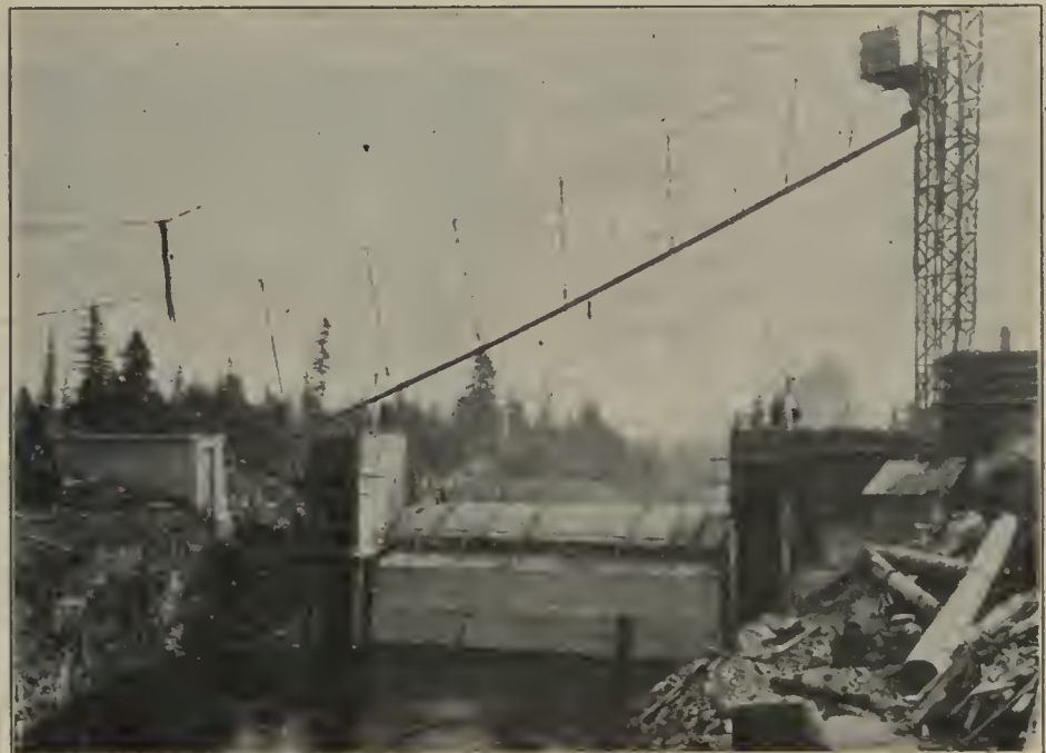
Easton dam, Kittitas division, Yakima project, Washington
