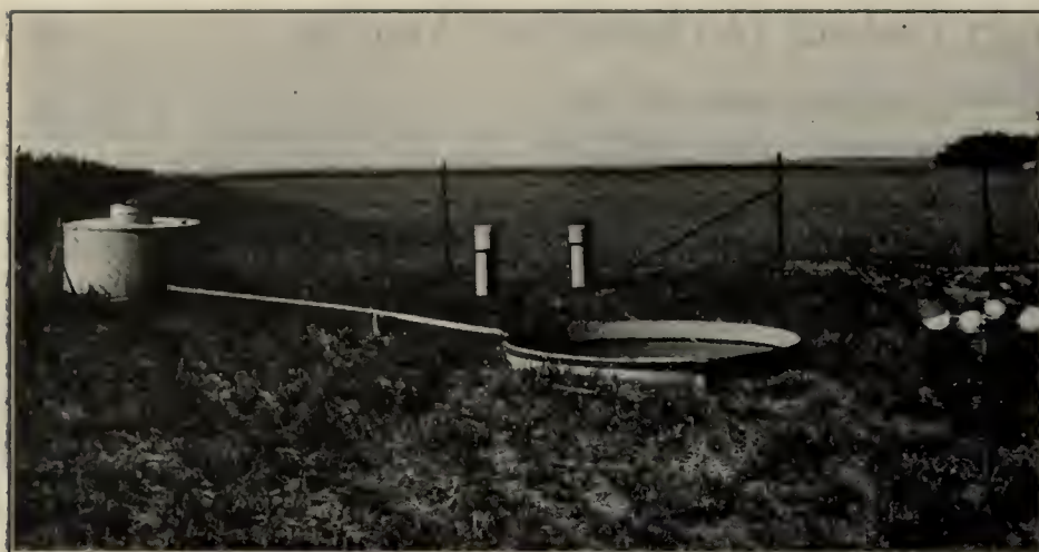
Land evaporation pan at Newell Experiment Farm, Belle Fourche project, S. Dak.
