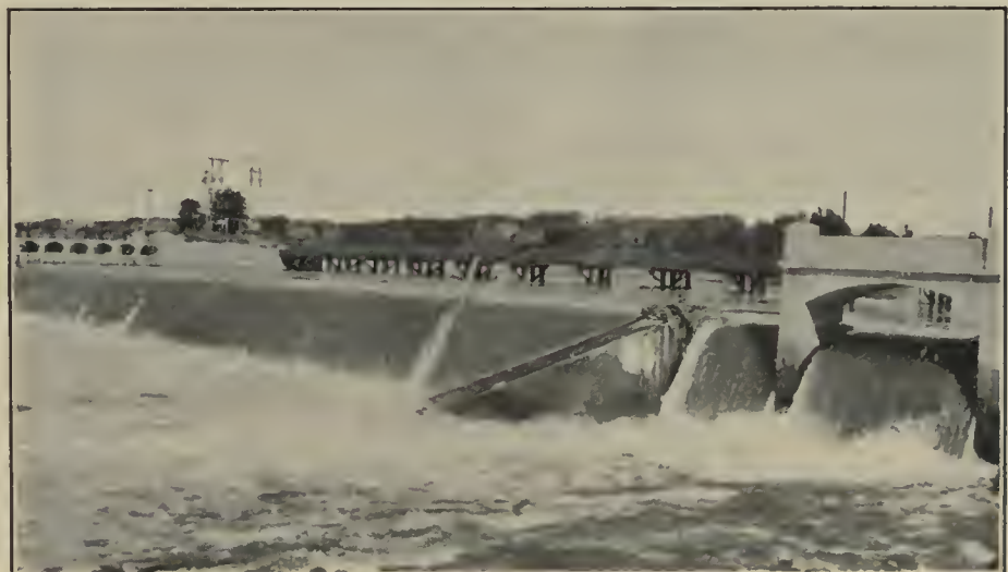
Whalen diversion dam, North Platte project, Nebraska-Wyoming
