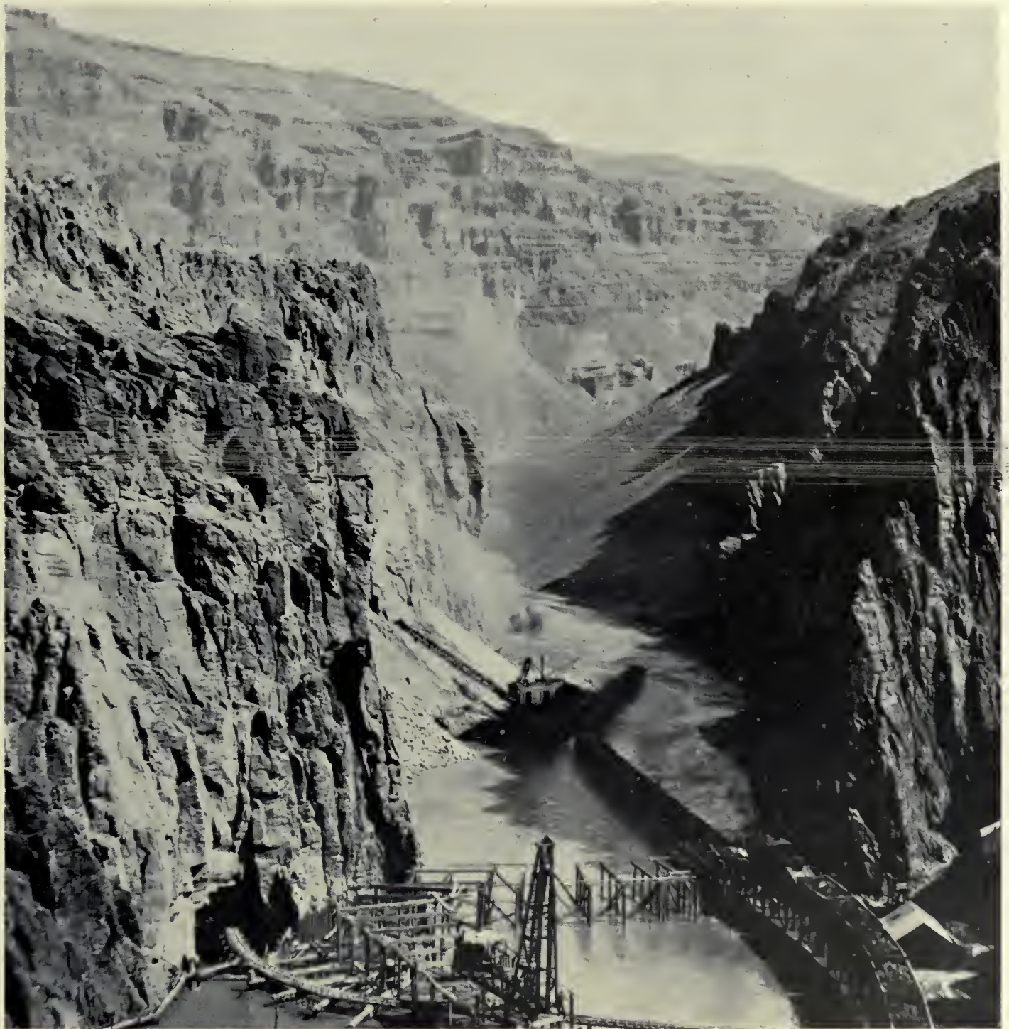
CONSTRUCTION PROGRESS ON 405-FOOT OWYHEE DAM
