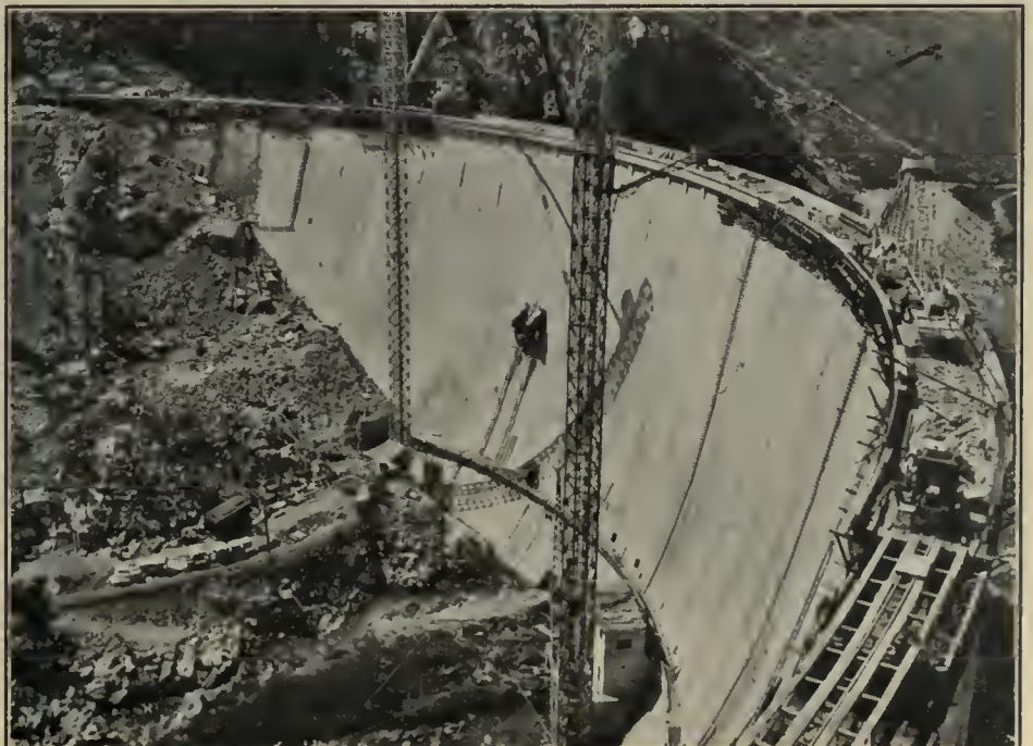
Gibson dam, Sun River project, Montana, nearing completion
