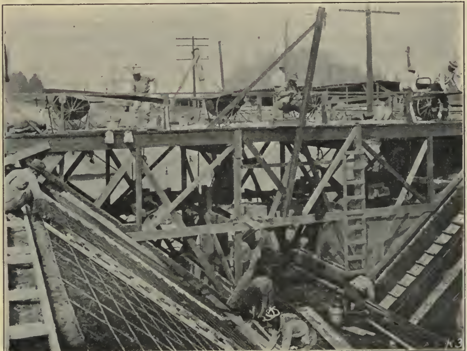
Apparatus used in placing concrete canal lining, Kittitas Main Canal, Kittitas division, Yakima project, Washington
