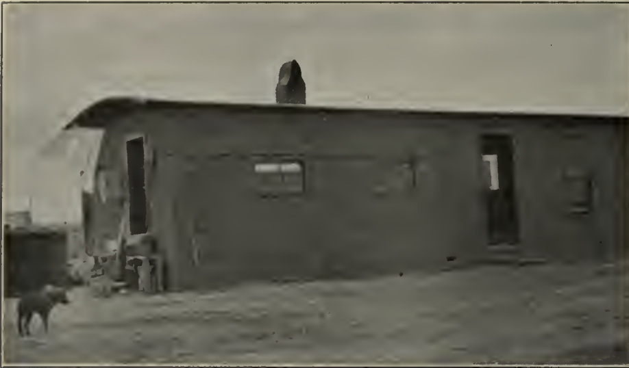
The adobe home of a new settler on the Willwood division, Shoshone project, Wyoming
