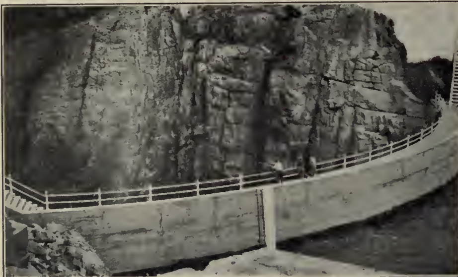
UPSTREAM FACE OF SHOSHONE DAM, WITH THE RESERVOIR FULL, SHOSHONE PROJECT, WYOMING
