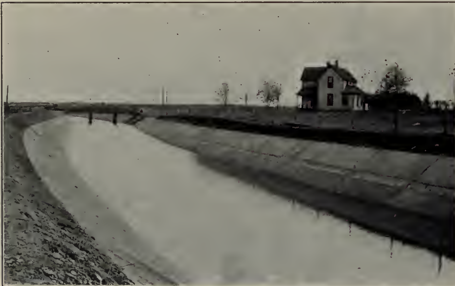
Main canal, Boise project, Idaho
