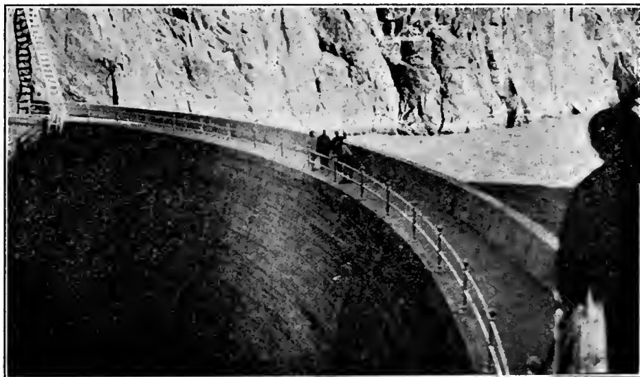
DOWNSTREAM FACE OF SHOSHONE DAM, SHOSHONE PROJECT, WYOMING
