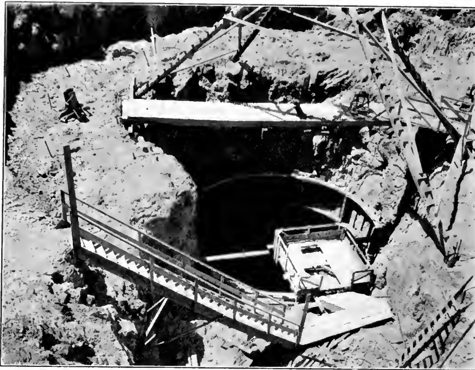
Glory hole at top of spillway shaft, Owyhee dam, Owyhee project, Oregon-Idaho
