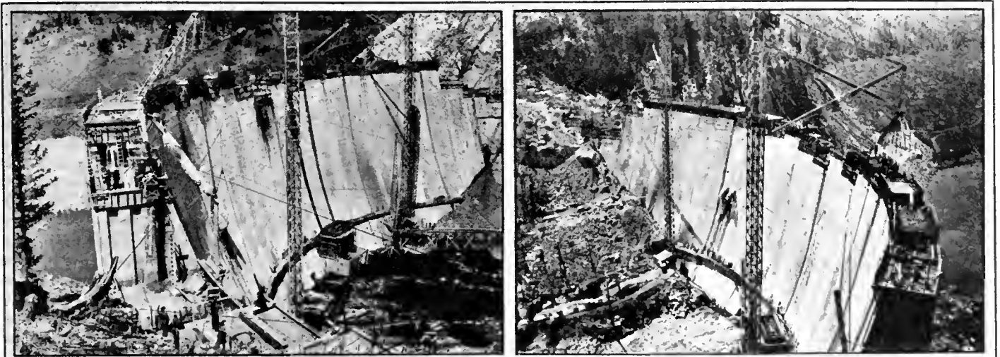
Gibson Dam Sun River project, Montana, nearing completion
