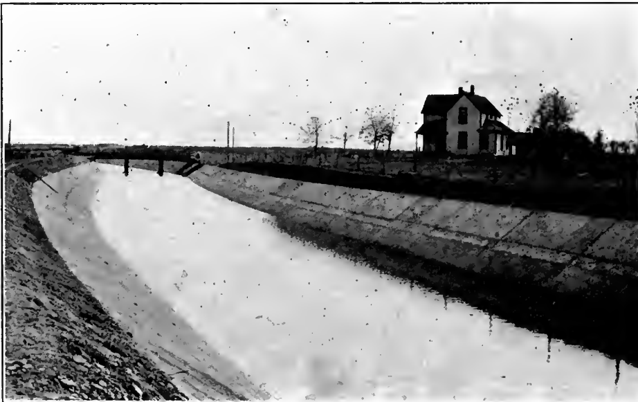
Main canal, Boise project, Idaho
