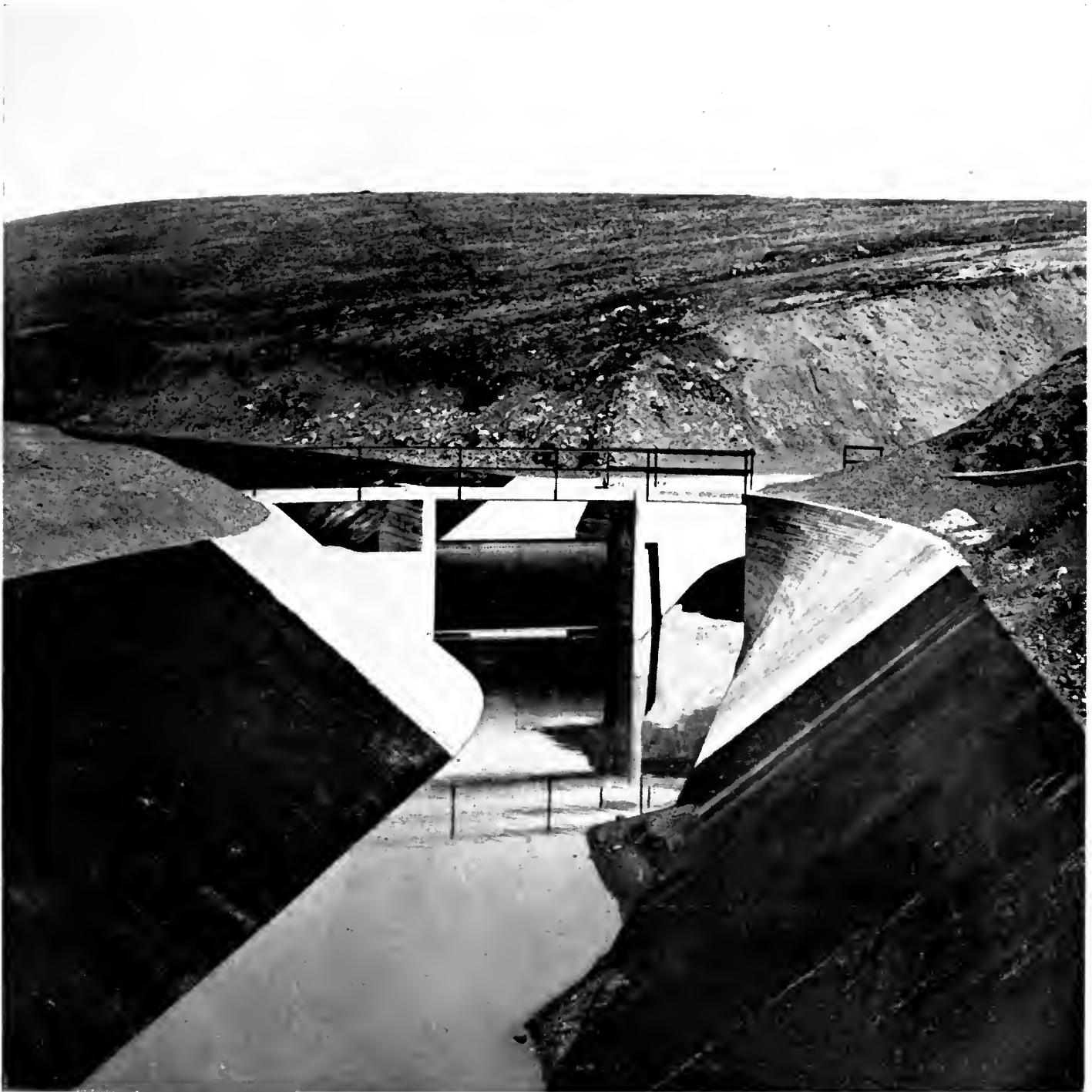
SOUTH BRANCH CANAL HEADWORKS, KITTITAS DIVISION, YAKIMA PROJECT, WASH.
