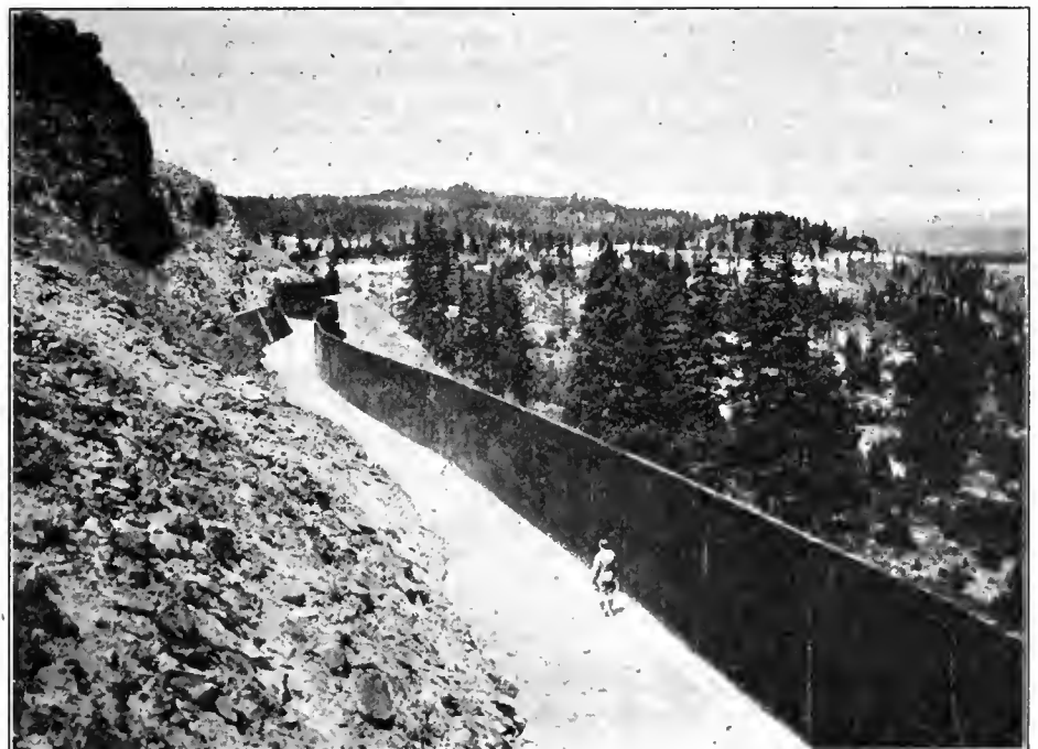
Combination section of Kittitas Main Canal, near Morrison Canyon, Yakima project, Washington
