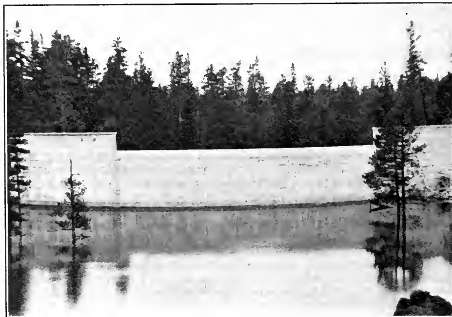
Gerber dam, Klamath project, Oregon-California
