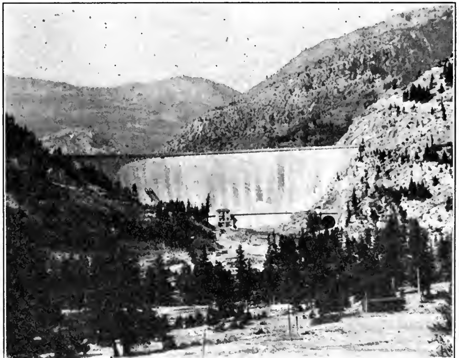
Gibson dam, Sun River project, Montana
