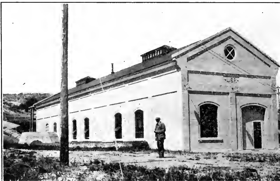
Dr. Alvin Johnson at the Lingle power plant, North Platte project, Nebraska-Wyoming
