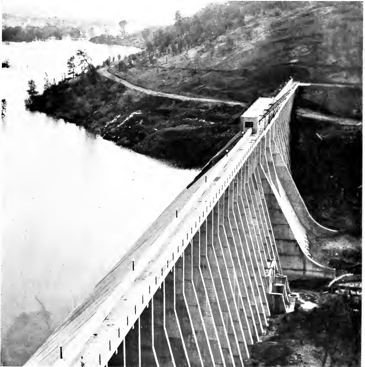
STONY GORGE DAM AND RESERVOIR FROM NORTH SIDE, ORLAND PROJECT, CALIFORNIA
