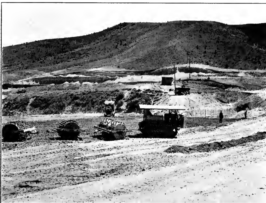
Tampers working on Echo dam fill, Salt Lake Basin project, Utah
