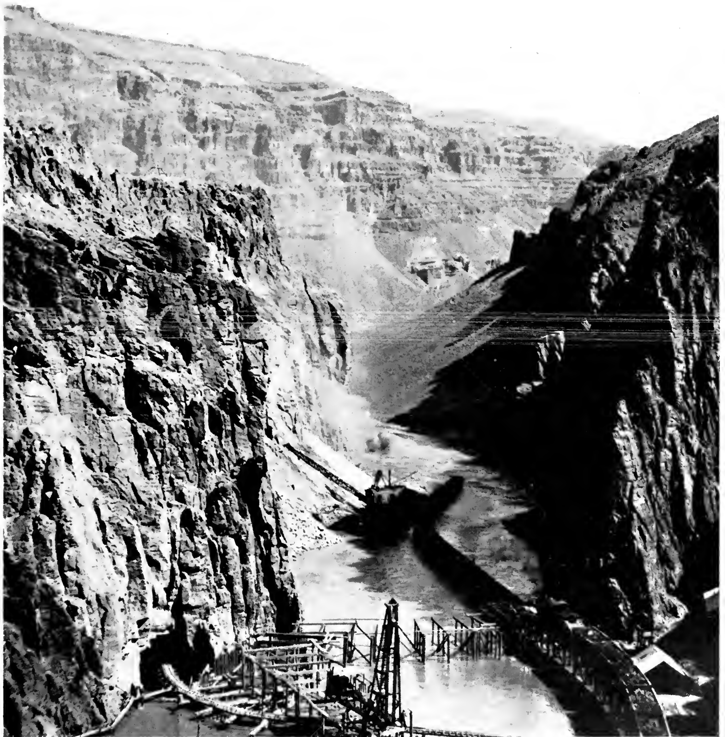
CONSTRUCTION PROGRESS ON 405-FOOT OWYHEE DAM
