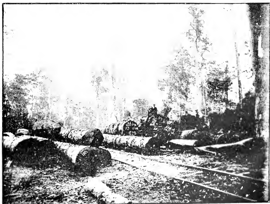
TALLOW-WOOD LOGS, BROUGHT FROM FOREST TO WHARF ON WOODEN TRAIN-RAILS, MANNING RIVER, NEW SOUTH WALES.
