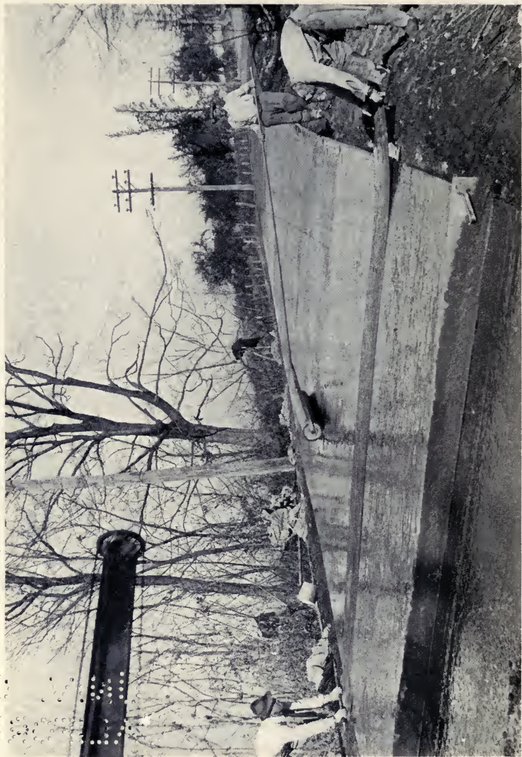
CONCRETE PAVEMENT FINISHING WITH STRIKE-OFF BOARD, CANVAS BELT AND ROLLER
