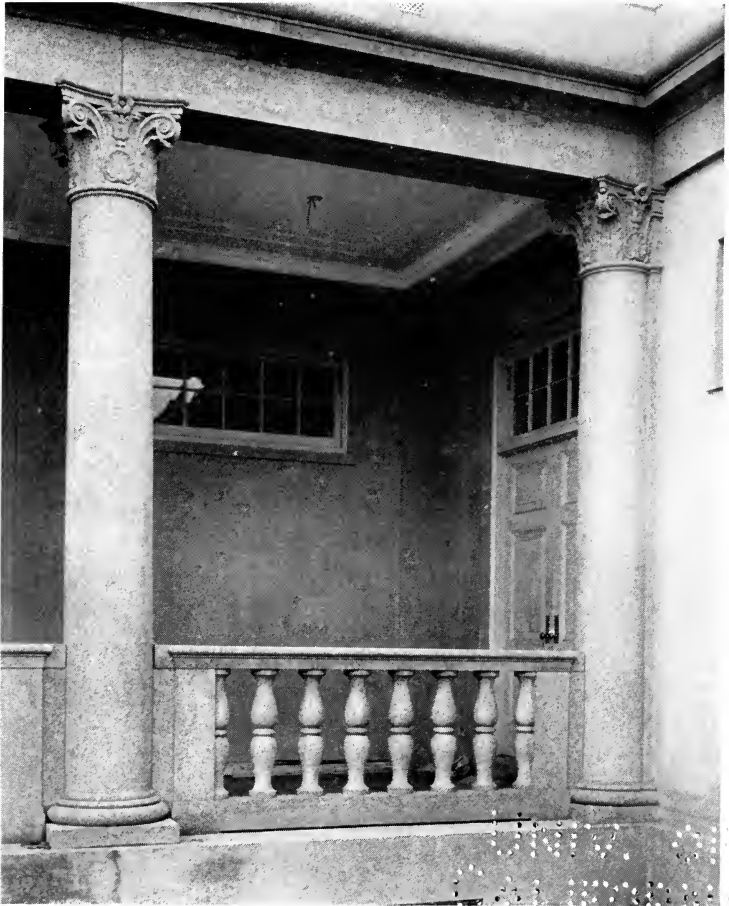
DETAIL OF SECONDARY PORCH, POTOMAC PARK FIELD HOUSE, WASHINGTON, D. C.
