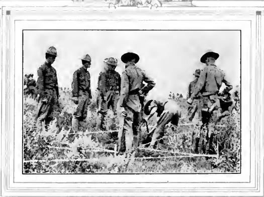
LAYING OUT TRENCHES WITH TAPE
