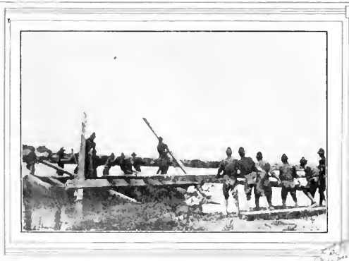
CONSTRUCTING PONTON BRIDGE
