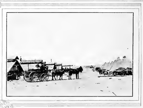
THE ENGINEER'S CAMP
