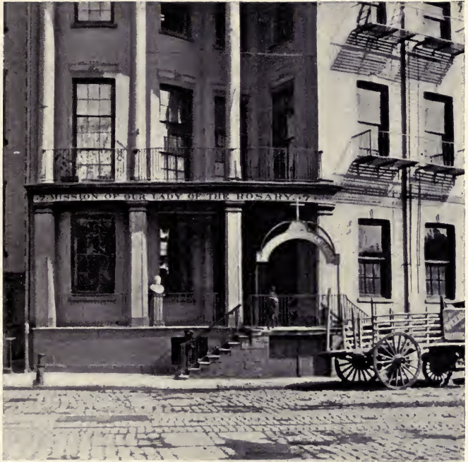
JACOB DOLPH'S HOUSE, NO. 7 STATE STREET. — BUNNER.
