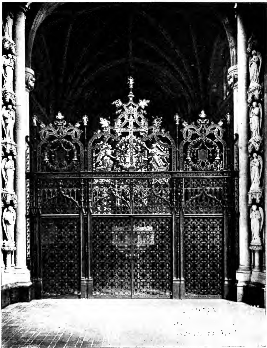
ENTRANCE GATE TO THE BELMONT CHAPEL, CATHEDRAL OF ST. JOHN THE DIVINE HEINS AND LA FARGE, ARCHITECTS (PAGE 374)
