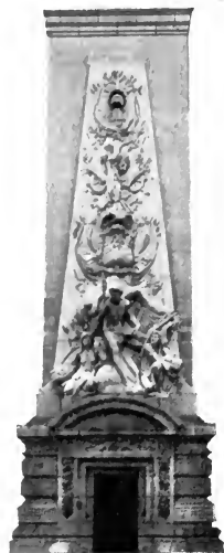
DECORATIVE PANELS "COMMERCE" CARL A. HEBER, SCULPTOR DETAIL MANHATTAN BRIDGE BOWERY TERMINAL
